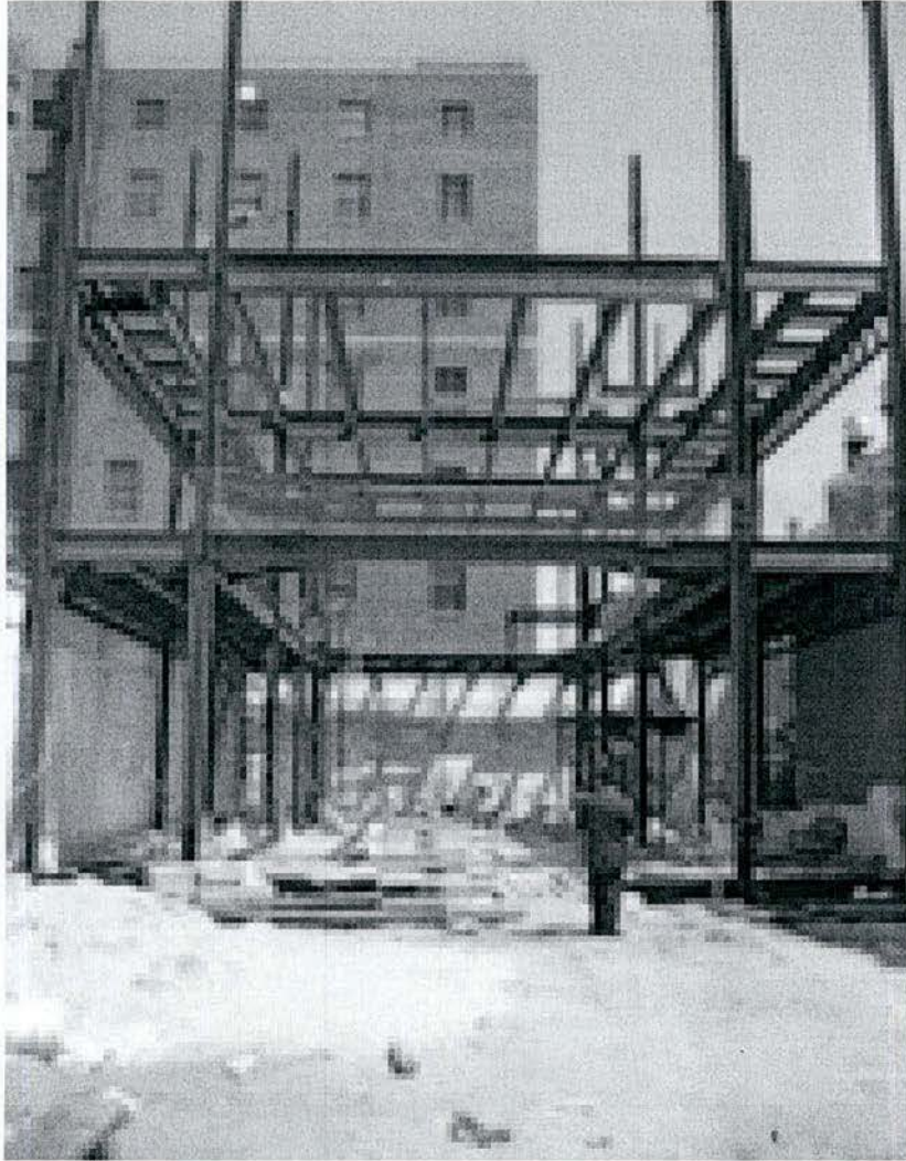
Figure 1. Boris Kandov standing in front of the construction site of the Bukharan Jewish Community Center in Forest Hills, July 2003.
