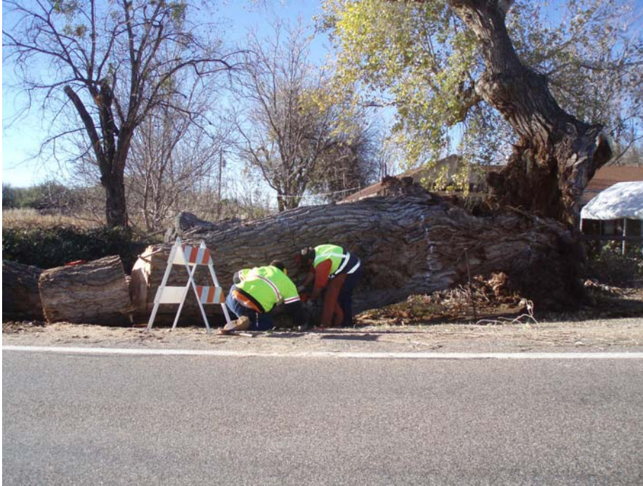
(Fig. 5, Country Brush Crew Hazard Tree Removal)
