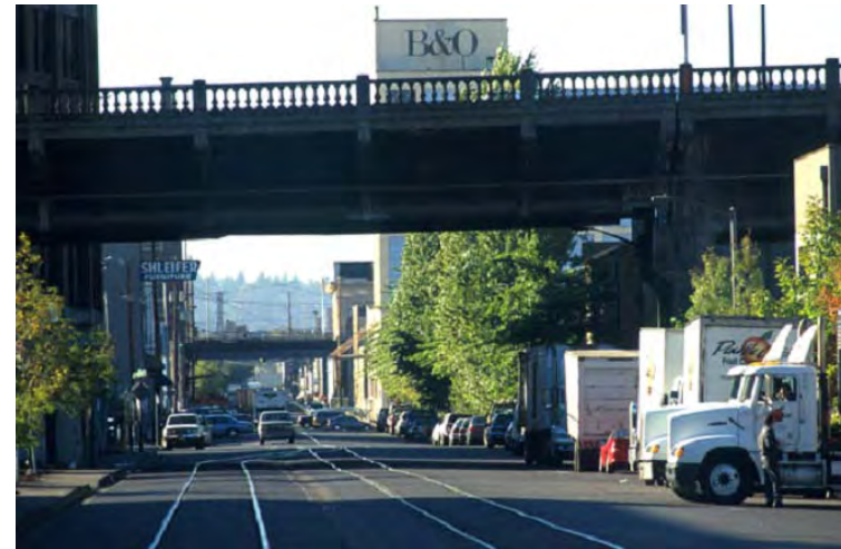
NE 3 rd Avenue looking south under the Burnside Bridge.
