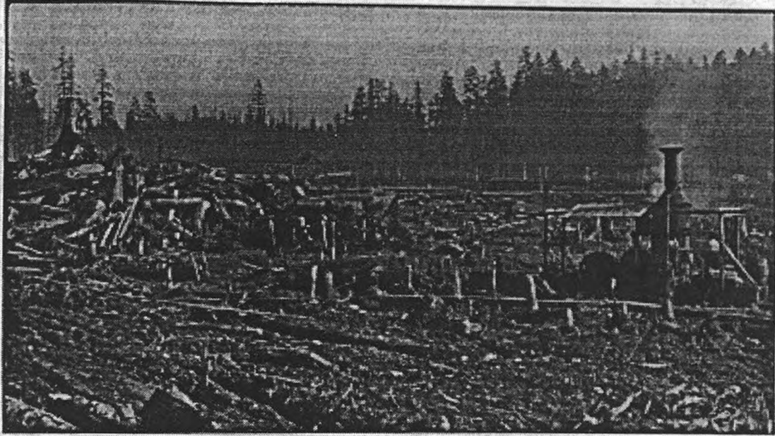
Filing Logs and Stumps with a Dooley Engine; much more rapid than the old way of burning in small piles.
