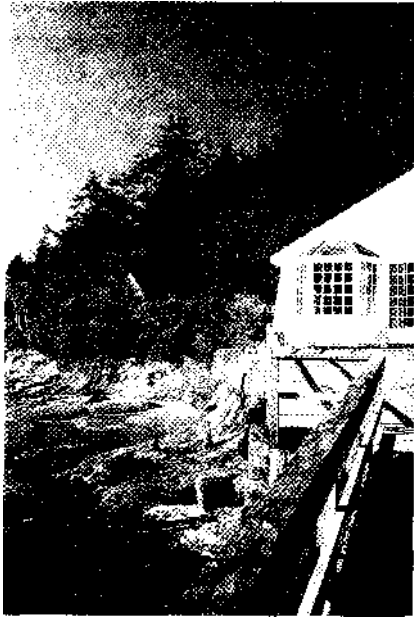
Fig. 2. The OIMB auditorium at Coos Head.
