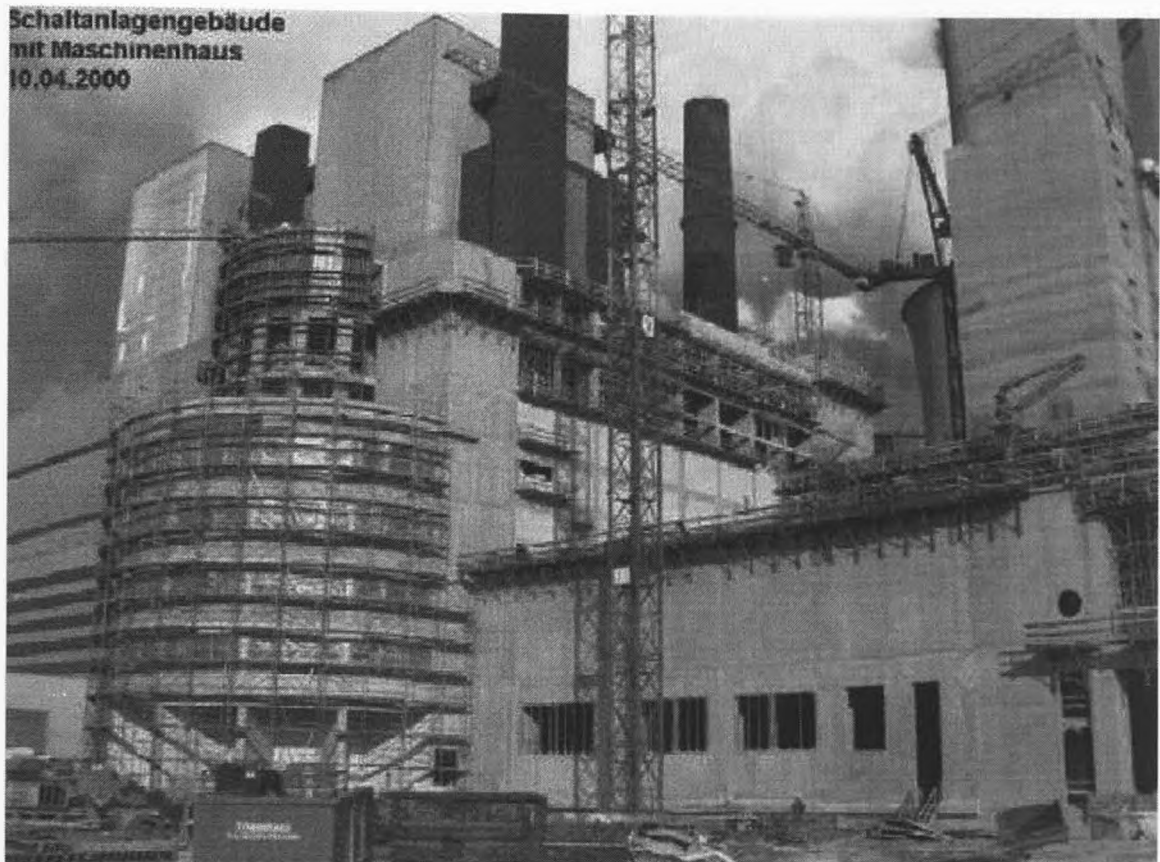
Figure 6. Rearview of coal power plant construction
