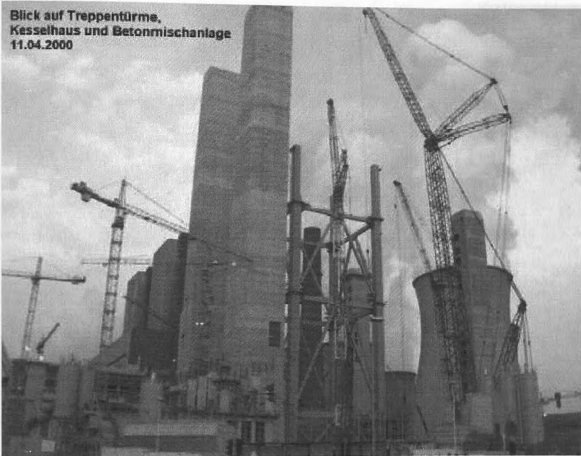
Figure 5. Construction of new high efficiency coal power plant: upper combustion area
