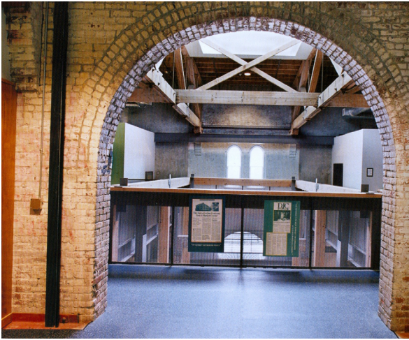
Interior reuse of building structure
