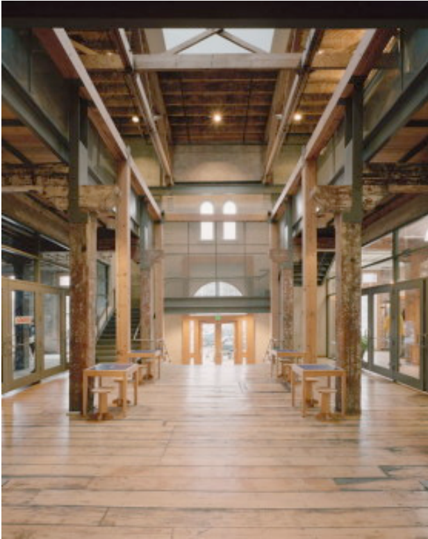
Central atrium space showcases the local heavy timber industry see in original structure of the warehouse
