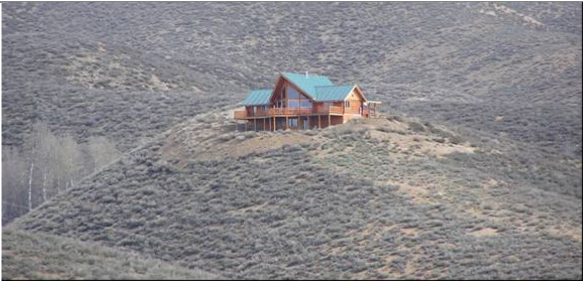
Figure 8. Soldier Mountain Ranch located on slope with heavy sagebrush fuel and limited survivable space.
