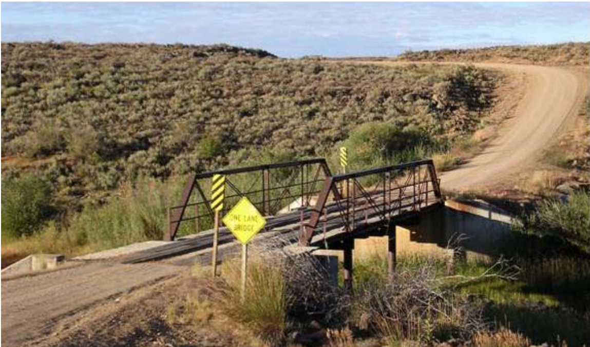
Figure 13. Five ton weight limit “restricted” bridge over Camas Creek.
