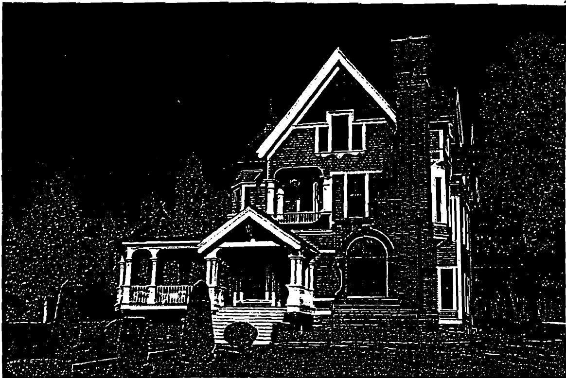
Nunan House - 635 North Oregon
