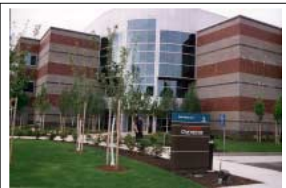
Landscaping can help buffer industrial impacts to adjacent properties.
