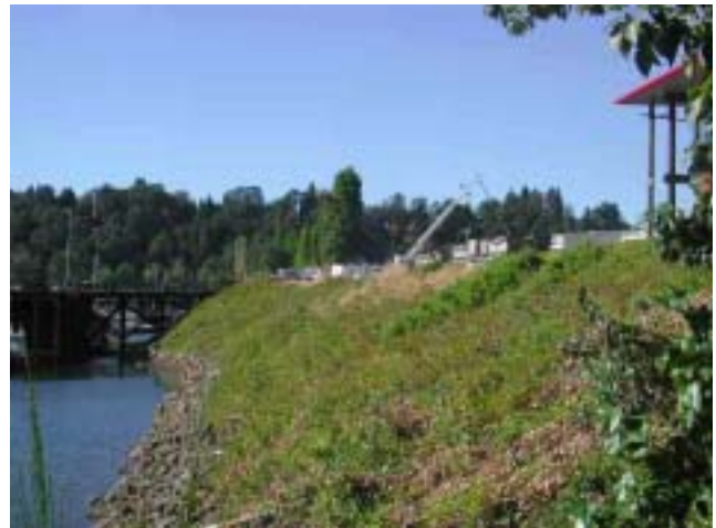
Bank constraints near N. Ensign (Port property)
