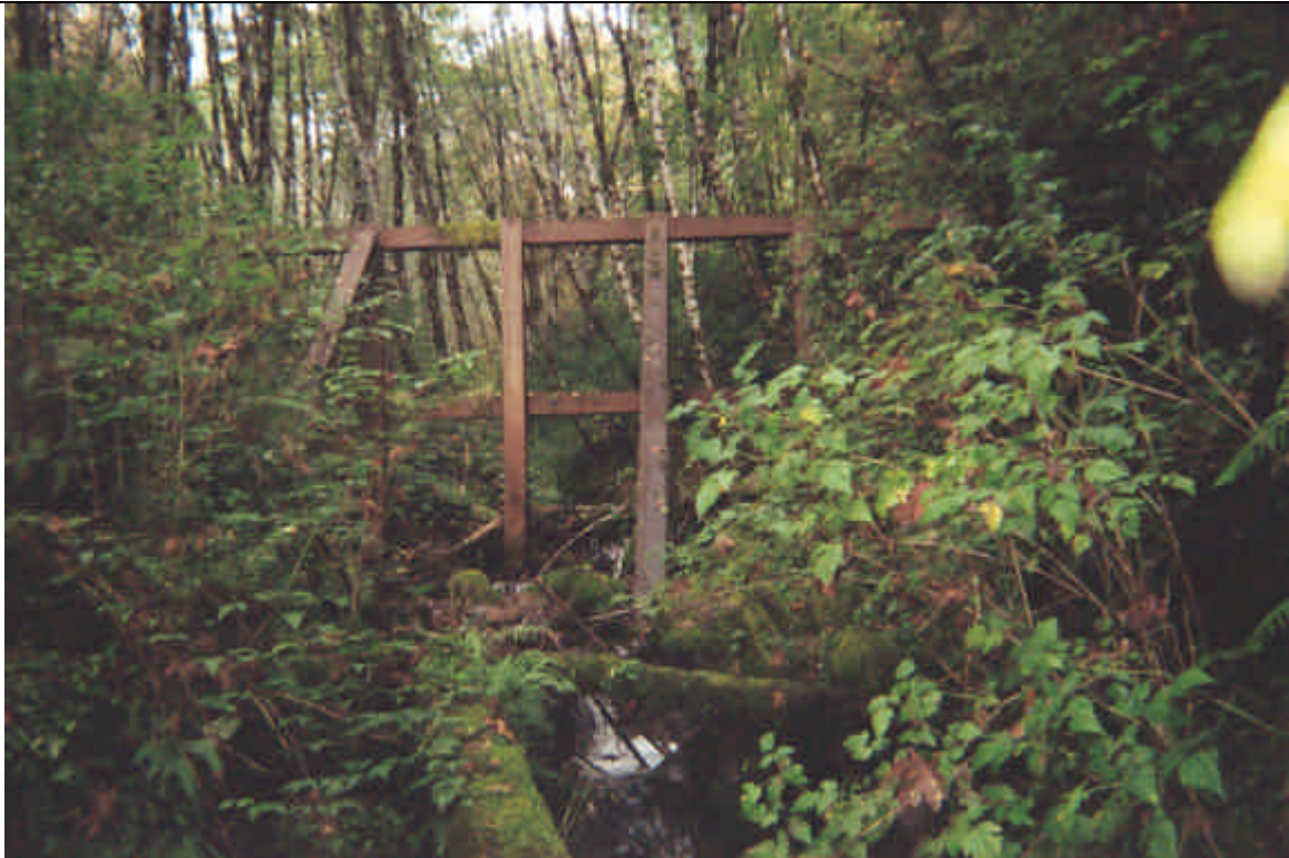
Photo 2: Downstream of trash rack looking upstream.
