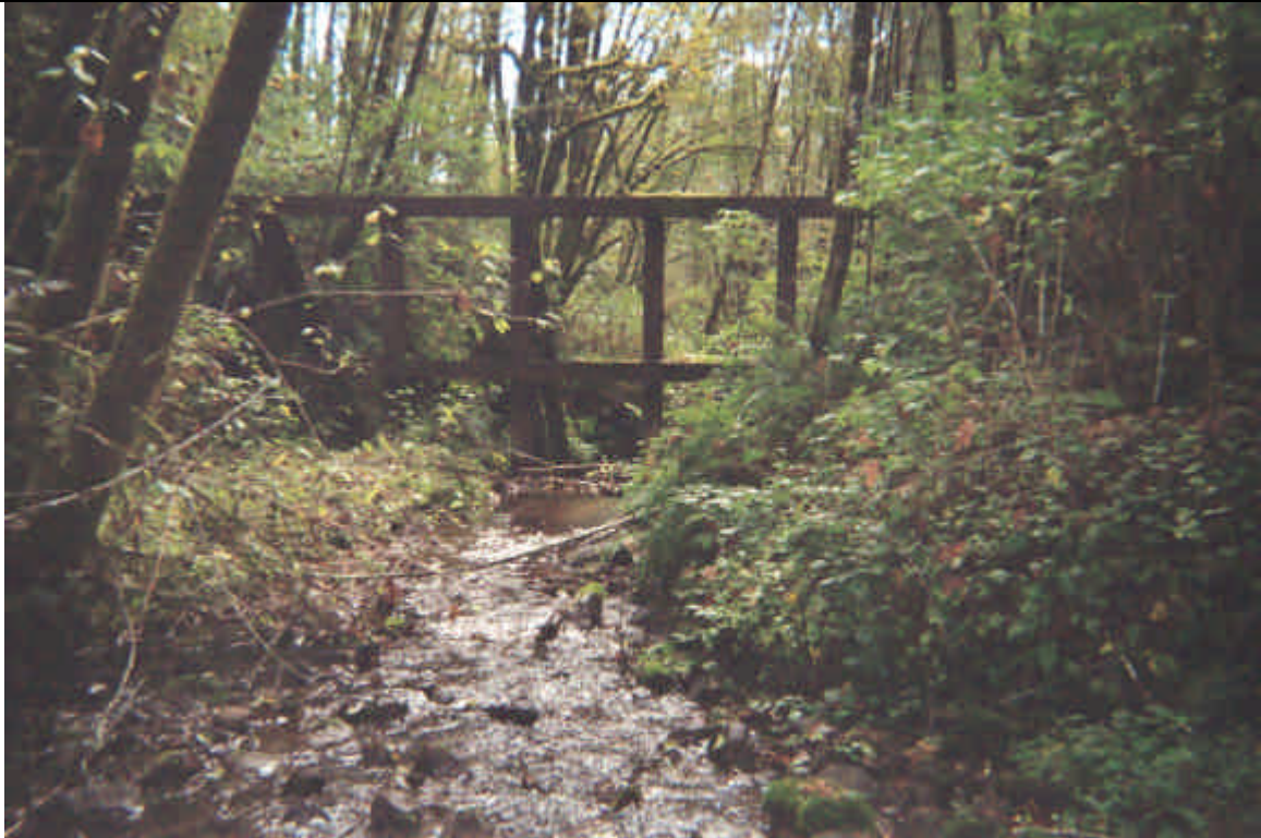
Photo 1: Upstream of trash rack looking downstream.
