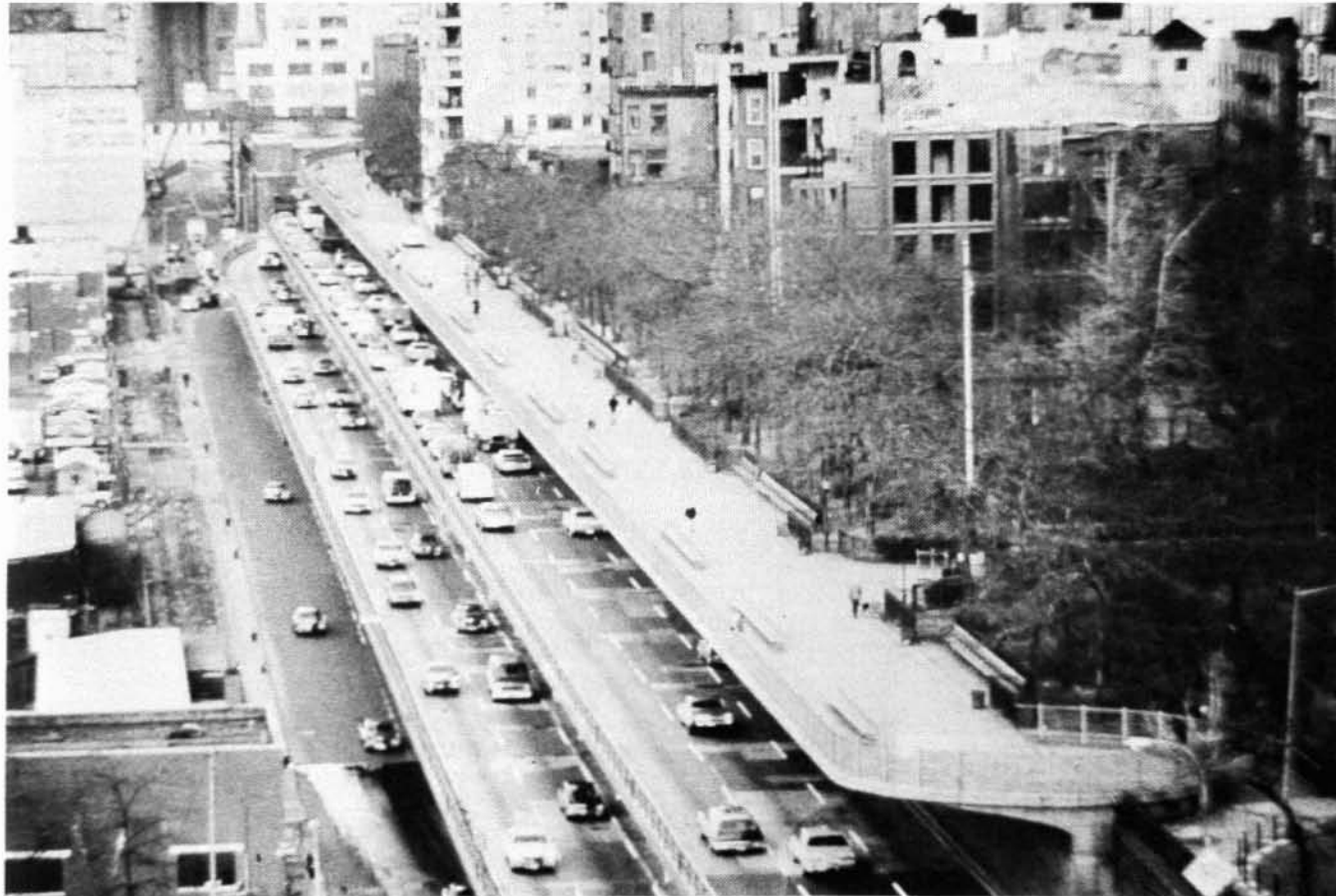
Brooklyn-Queens Connecting Highway at Brooklyn Heights, New York.
