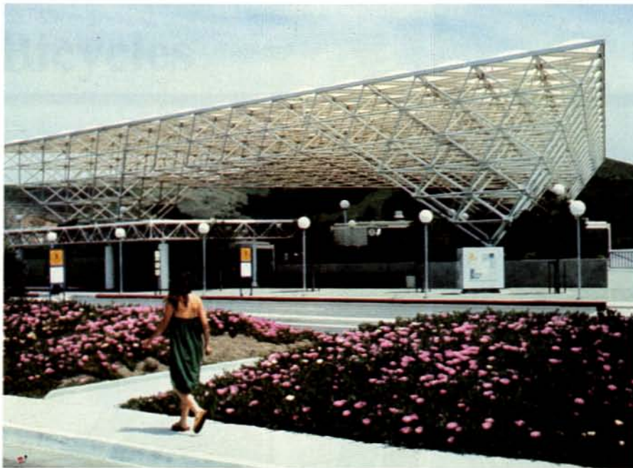
a. Space frame structure is easily seen from the boat.
