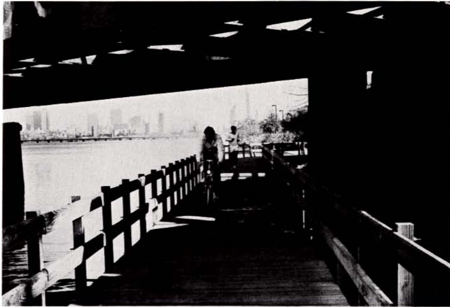
a. Bikeway under Boston University Bridge.
