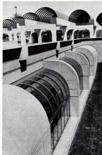
c. Excavation allows for windows at the platform level.
