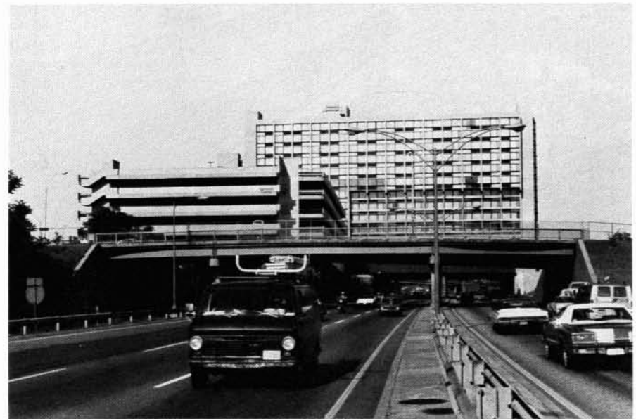
Hotel in Newton, MA., built on air rights over the Massachusetts Turnpike.
