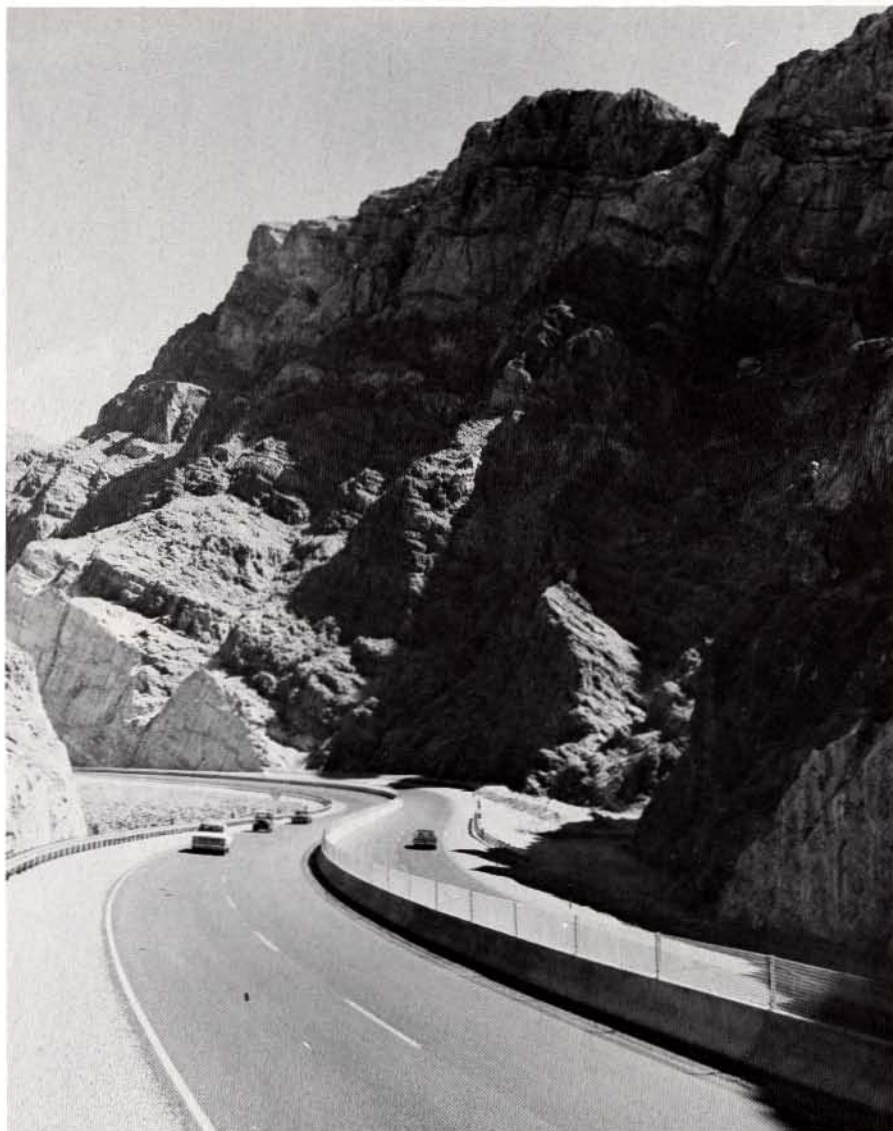
Roadway elements underscore drama of canyon route.
