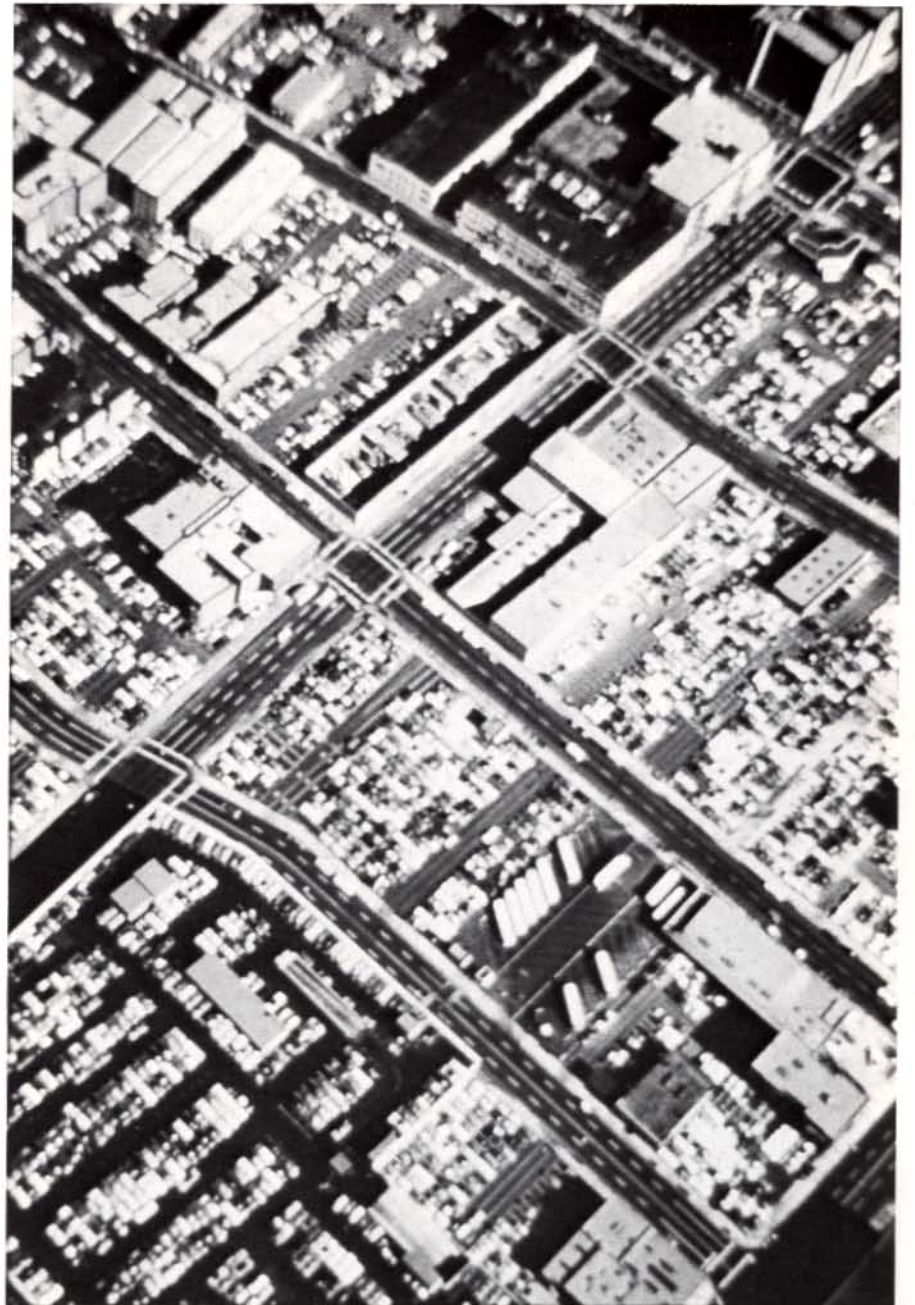
c. Vacant lots used for parking erode the urban streetscape.
