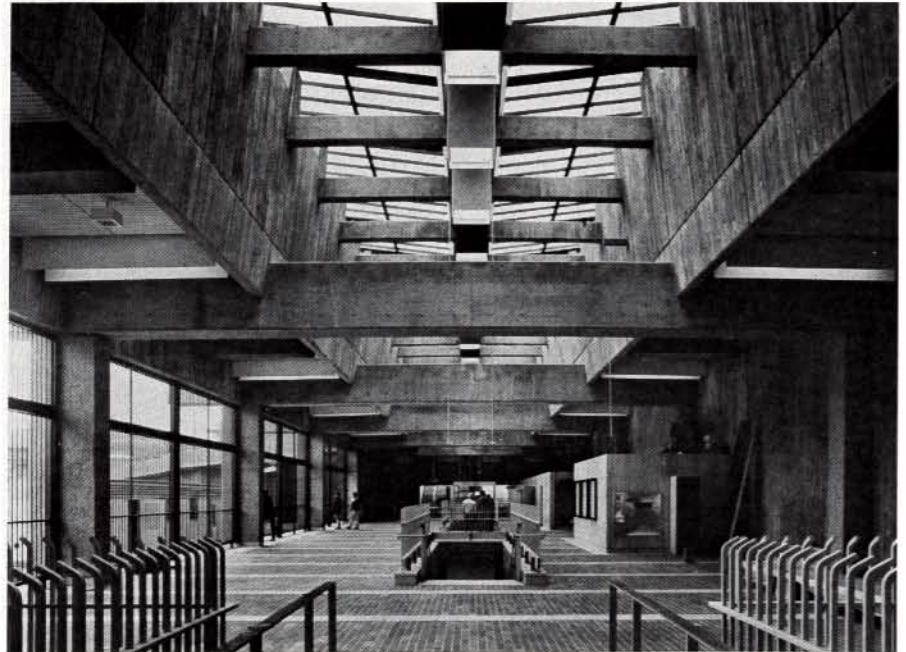
a. Design of BAKI Glen Park Station employs standard system elements in a distinctive way.
