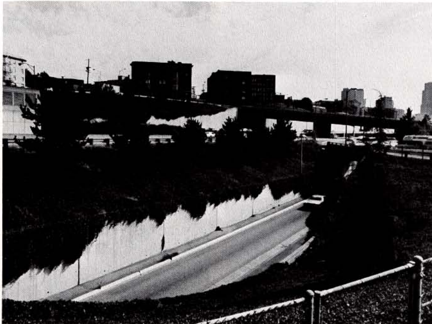
c. Greenery enhances retaining walls. Seattle.
