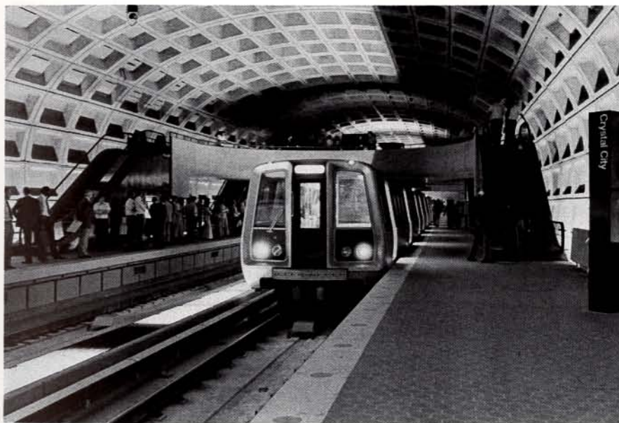
a. Typical station. Washington METRO.
