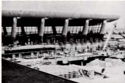
d. Terminal expansion under construction.
