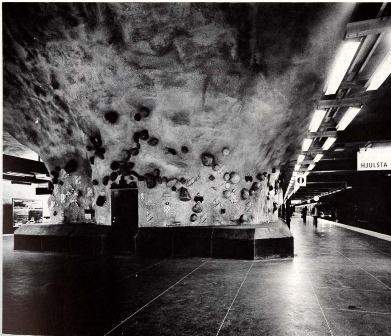
Stockholm subway tunnel has been designed to retain its cavelike walls, with artistic interpretations at each station.
