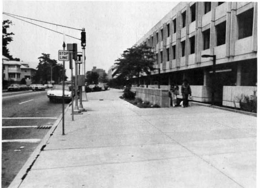
b. Parking garage forms a wall on residential side.
