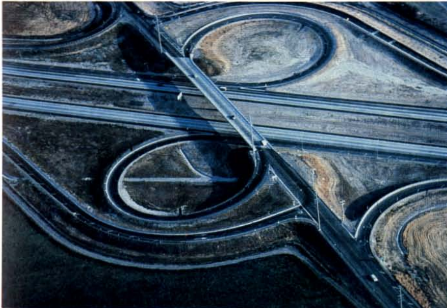
a. Highway interchanges leave behind hard to use land
