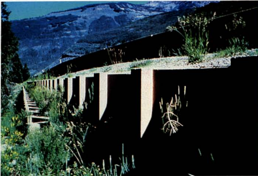
a. Tiered, reinforced earth retaining walls before planting with grass.
