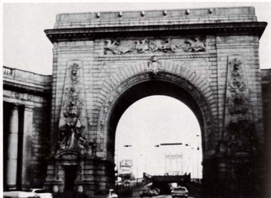
a. Bridge portal, New York.
