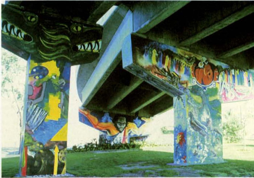
a. Murals under freeway, San Diego.
