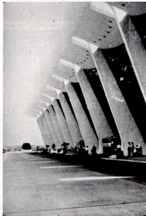
b. Colonnade at terminal entry.
