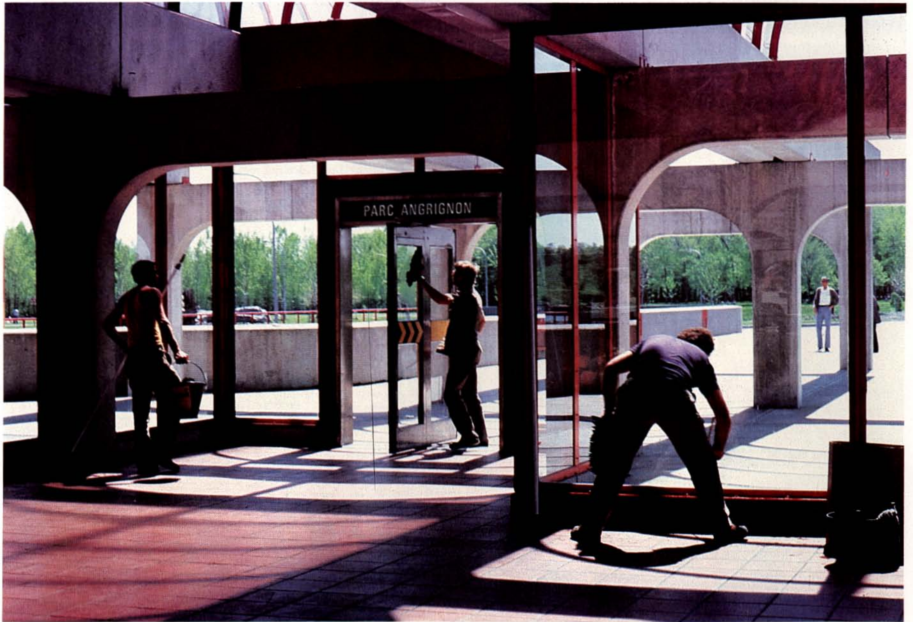
Maintenance crew at work.
