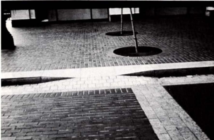
a. Paving detail, Market Street, San Francisco.
