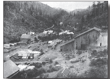
The Blewett Mines in 1905. Originally called the Pesbastin Mining Camp. The large building on the right was a twenty stamp mill used to process gold ore. All material needed to build the camp had to come from Ellensburg or Cle Elum over Blewett Pass.
