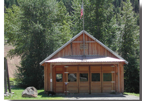
Liberty Fire Hall. The community hall is still under construction in the summer of 2004 and was used for the initial public meetings to discuss the fire plan.
