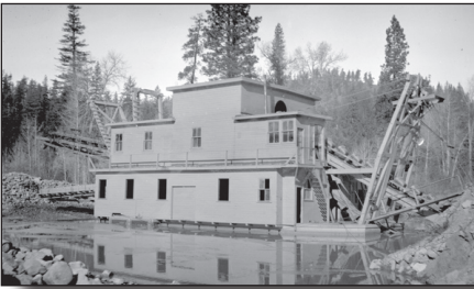
Swauk Gold Dredge in 1926. This large gold dredge, the Powder River Gold Dredge No. 2, was brought in from Sumpter, Oregon, in 1925. It started working in the Swauk at the big rock outcrop north of Liberty Cafe and got just up Deer Gulch before being stranded. It could not handle the hard, shallow bedrock. The dredge was dismantled and shipped to Alaska, the barge it sat on still rots in the dredge pond in Deer Gulch.
