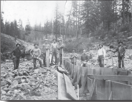
Early Mining Flume Near Liberty. The flume was used for placer mining where gravel from a stream bed is washed to recover the gold.
