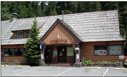
Mineral Springs Restaurant on Highway 97. The restaurant is on land leased from the Forest Service. The building is the old Swauk Recreation Lodge built in 1940 and later moved to its present location.
