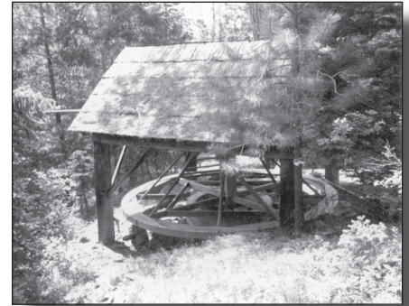
Virden Arrastra in the 1970's. The arrastra was used to grind gold ore. The arrastras around Liberty used a horizontal undershot water wheel for power, probably the only place in the world to do so. Vandals destroyed the arrastra in 1974. A working replica of the Virden arrastra was built in Liberty in 1974.
