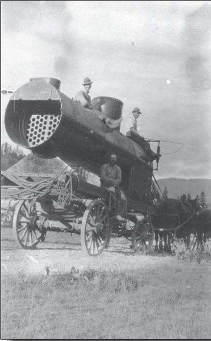
Hauling a Boiler for the Peshastin Stamp Mill. The miners had to build the wagon road over old Blewett Pass to haul large equipment from Cle Elum and Ellensburg for the stamp mill at Peshastin. That wagon road later became Highway 97.
