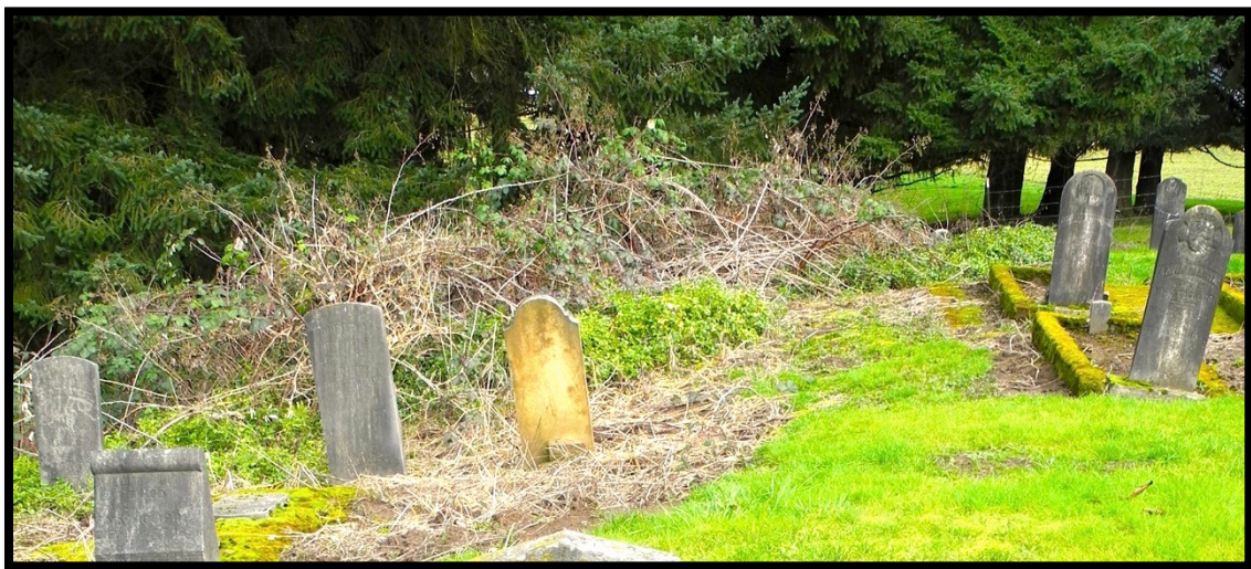
Figure 8.7 Eastern view toward the Northeast corner of Section I. Note the significant growth of vegetation, left , encroaching into the northern edge of many of these rows of interments, obscures some graves' above-ground components. (photo: author, 2012)
