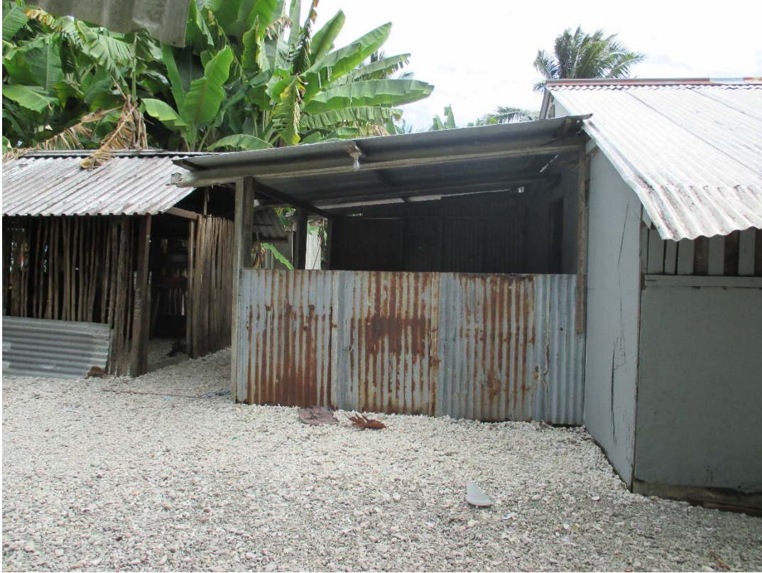
Figure 256. Photograph of cookhouse attached to house 'C'.
