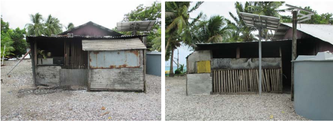
Figure 233. Photograph of cookhouse added onto House A
