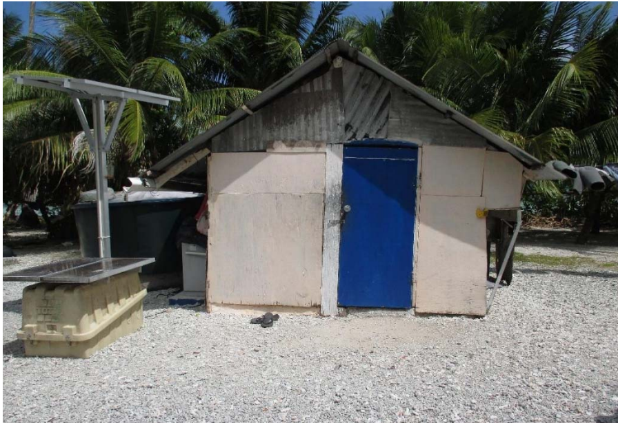
Figure 139. Photograph of a house constructed from recycled corrugated metal and plywood. The framing is a mix of dimensional lumber and local wood.
