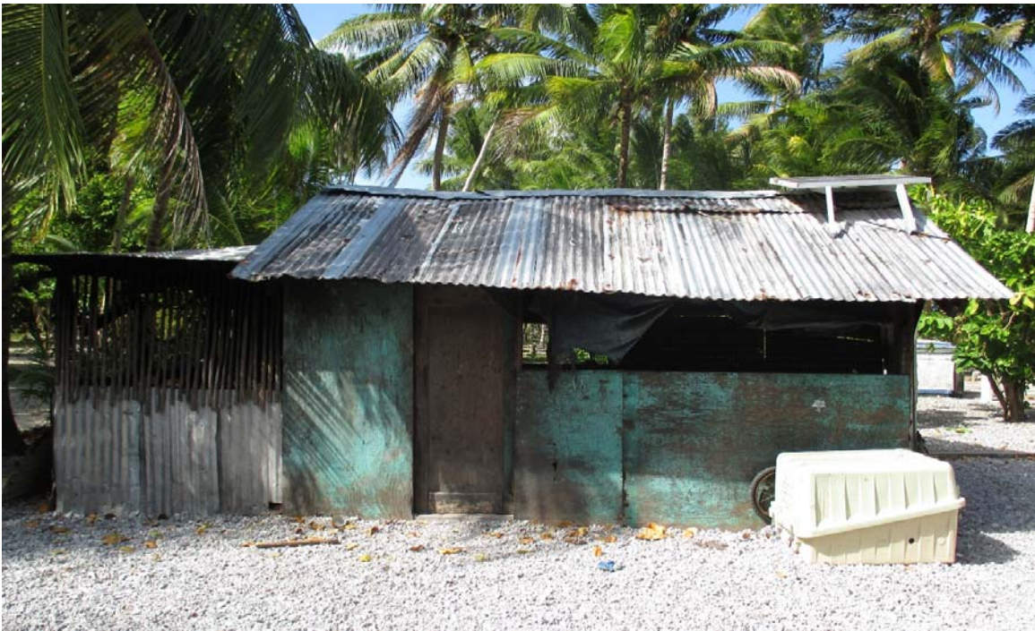
Figure 189. Photograph of entry facade to cookhouse on Monwat.
