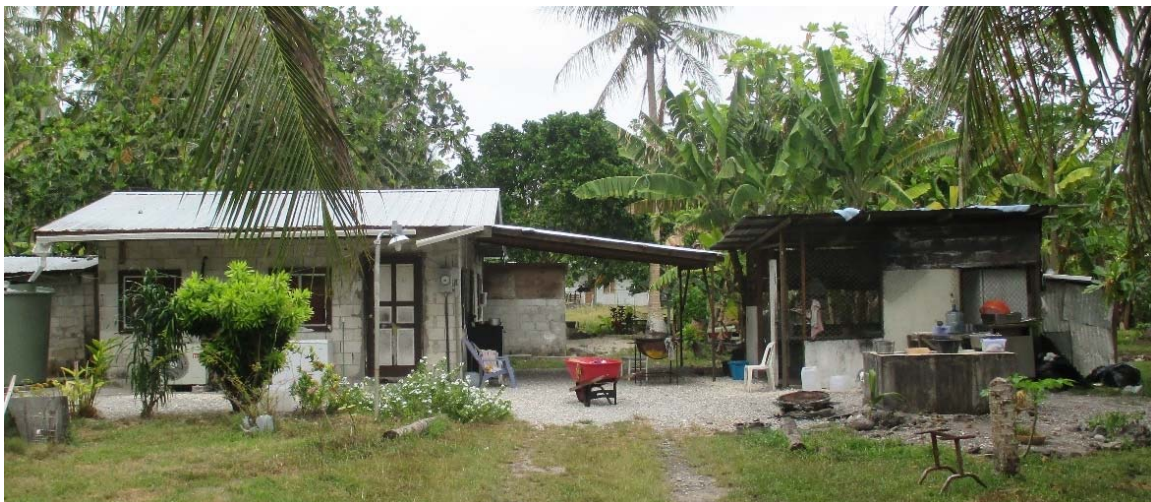
Figure 110. Photograph of the front of the house and cookhouse, showing the breezeway created between the two. The breezeway is the most used space.
