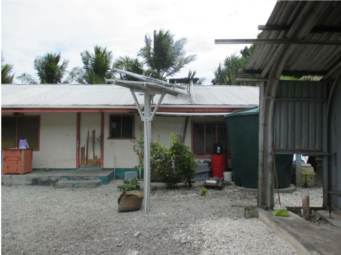
Figure 251. Photograph of house of the mayor and alap of Mojero. The material from a former Quonset hut can be seen to the right, which houses the virgin coconut oil processing facility.
