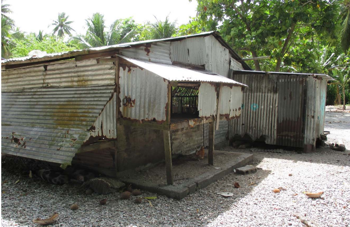
Figure 174. Photograph of the rear side of the cookhouse, showing the shelf and vent.
