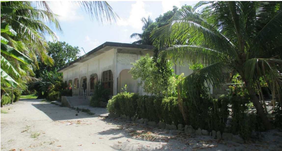
Figure 36. Photograph of the shophouse built on leased land on Moneibel wēto .
