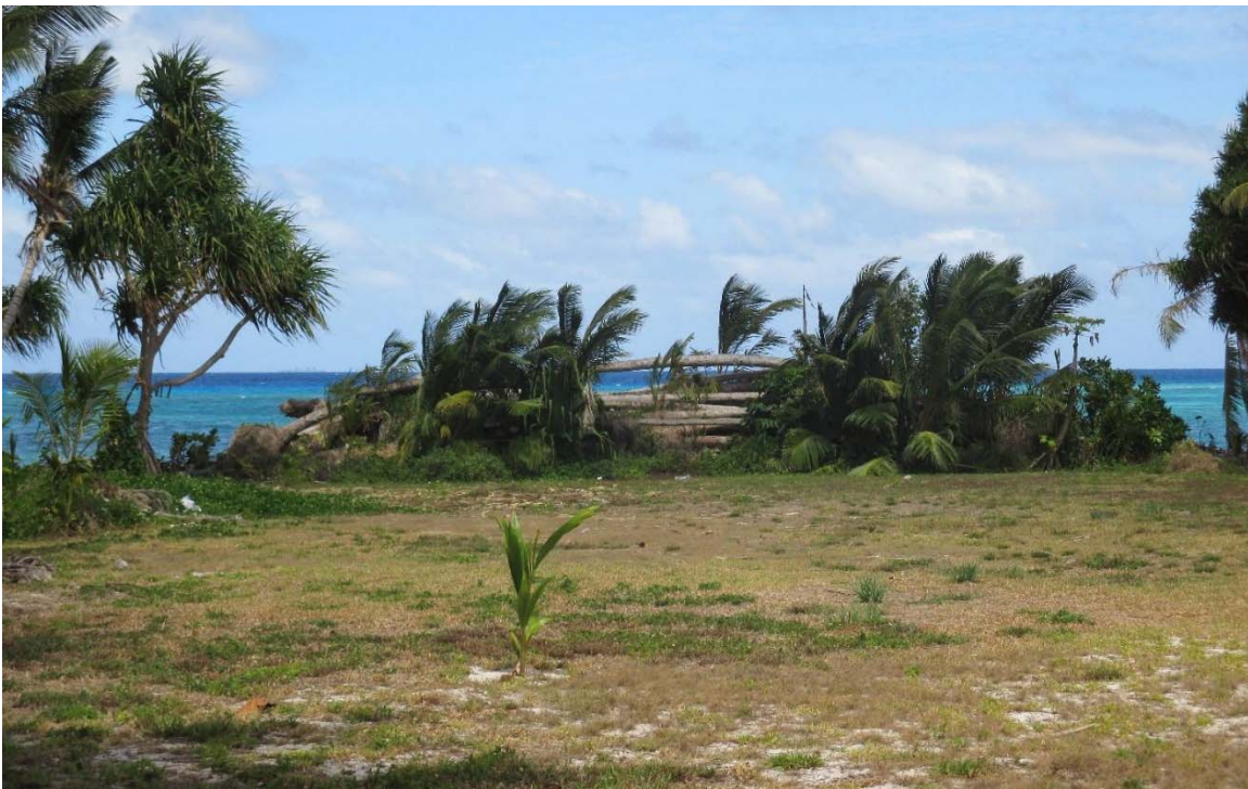
Figure 142. Photograph of a large berm created in Laura using coconut trees and rocks.
