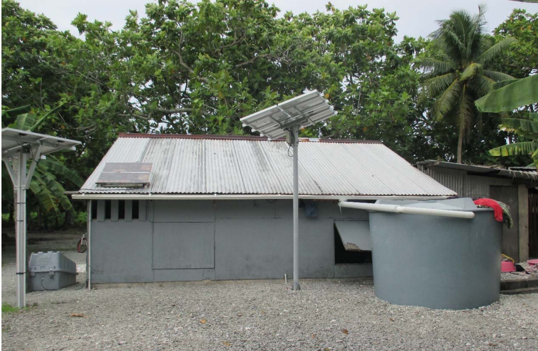
Figure 254. Photograph of east facade of house 'C'.
