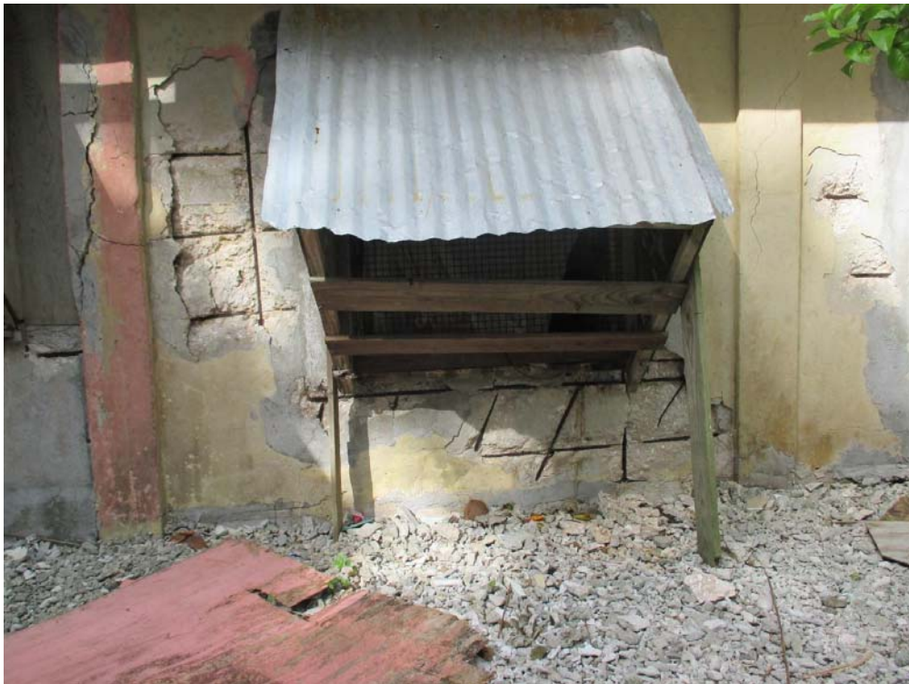
Figure 138. Photograph of a weather hood vent constructed in place of a window on the lagoon side of a house on Moneibel wēto , Namdrik.
