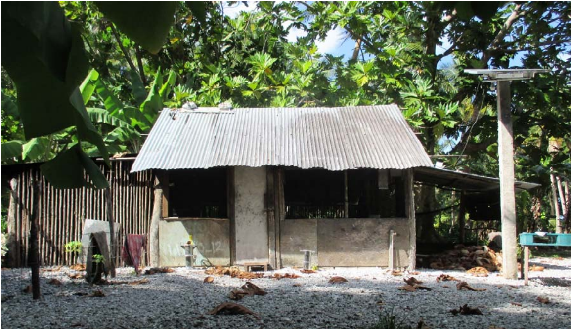
Figure 200. Photograph of the cookhouse of house 'C'.
