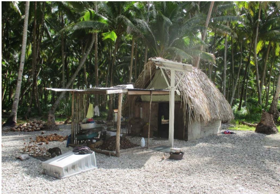
Figure 140. Photograph of a thatch house. The house has a mixture of materials used in its construction including traditional thatch, plywood, and canvas.
