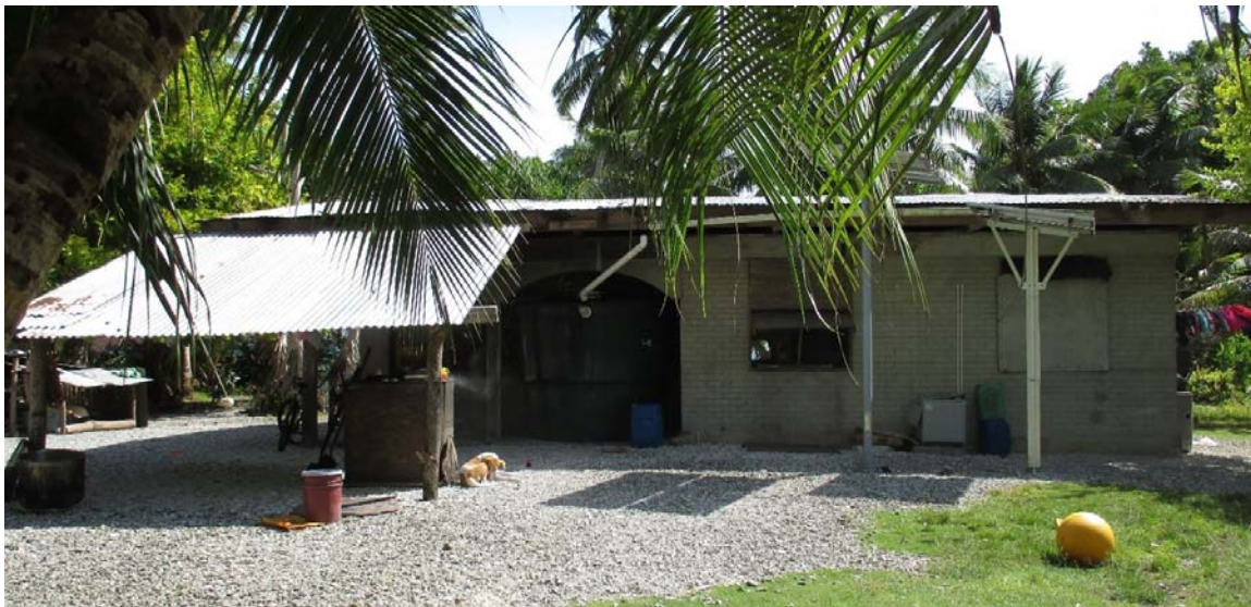
Figure 163. Photograph of house on Wijlang that was constructed in a Pohnpeian style. Notice the striked lines to resemble brick.
