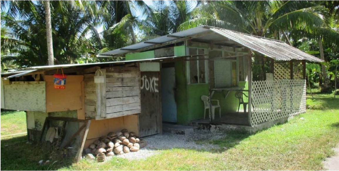
Figure 143. Photograph of a shop and cookhouse. Both are constructed from recycled material.
