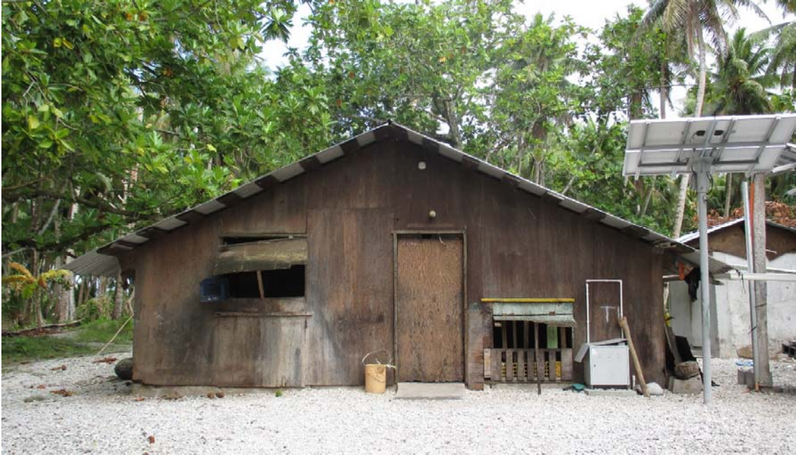
Figure 181. Photograph of ocean facing facade of house 'D'.
