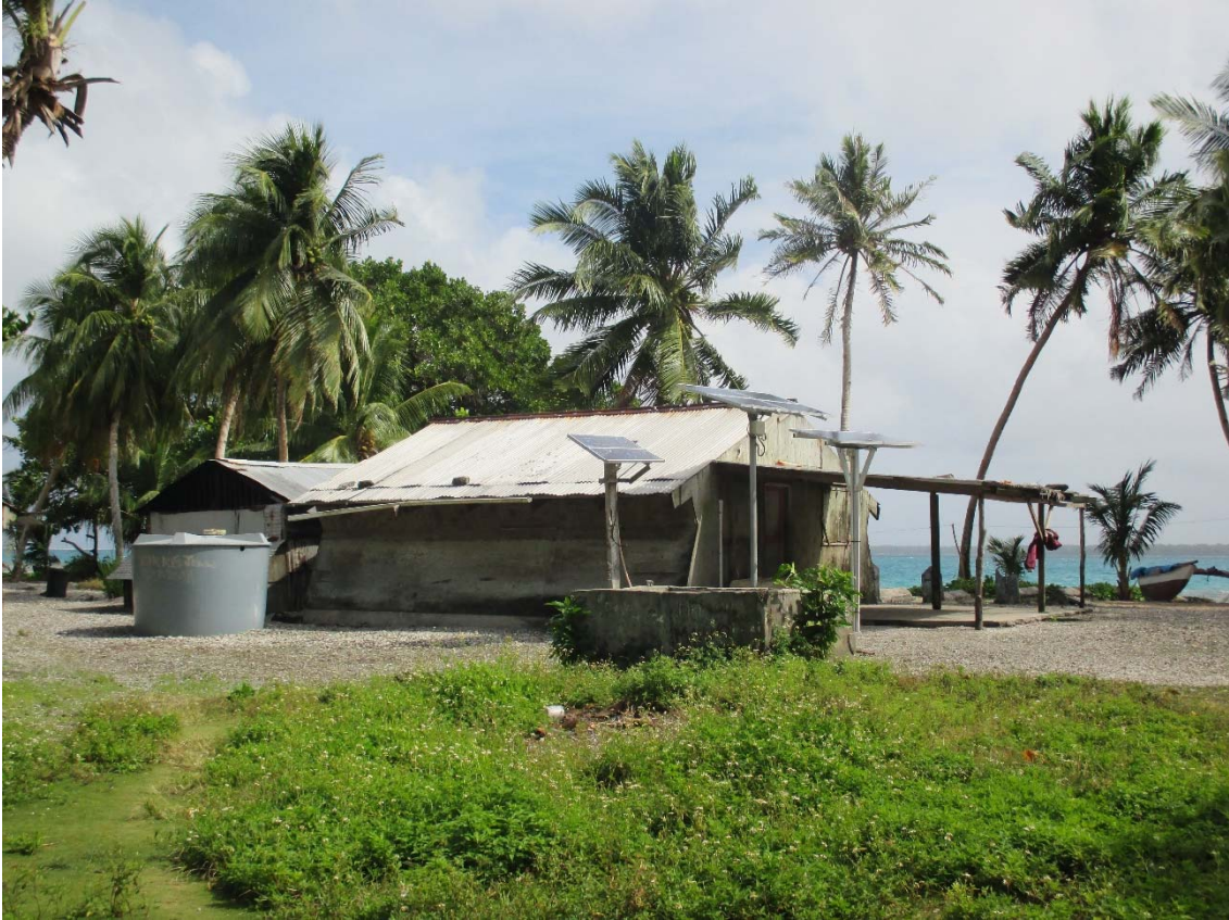
Figure 242. Photograph of house 'E' showing south facade.
