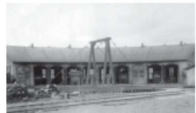
Historic roundhouse used to turn-around and repair train engines.
