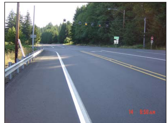
Eastbound US 20 Approach
