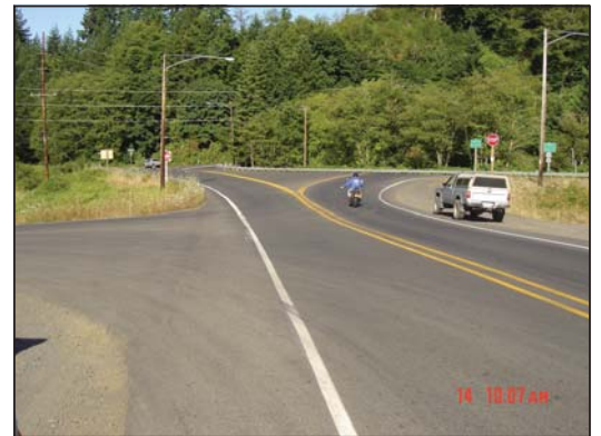
Northbound Business 20 Approach
