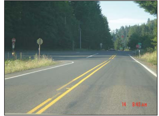
Southbound OR 229 Approach
