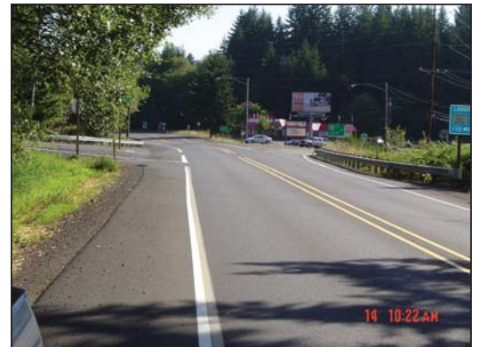
Eastbound US 20 Approach
