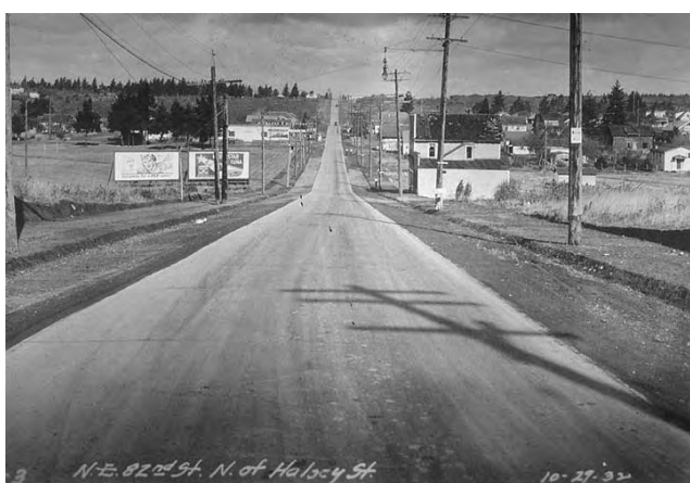
NE 82 nd , north of Halsey, looking north from where the Banfield Freeway is now, 1932. City of Portland photo
