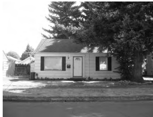
Modest house constructed in 1944, SE 88 th and Alder
