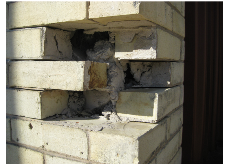
Brick missing from facade
