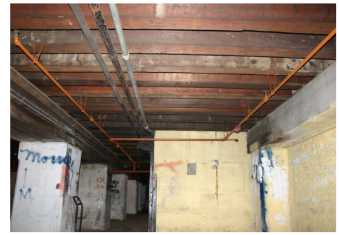
B. Existing Basement Conditions
