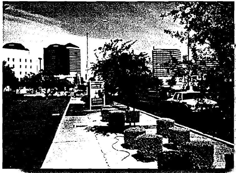
Thomas Road "After": A buffered lateral separation provides a better ("Level of Service "B") walking environment under the same traffic conditions.
