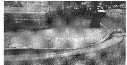
In the past, many corners in Portland were built with a single diagonal ramp.
