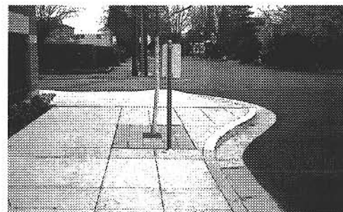
Curb extensions can shorten crossing distance.
