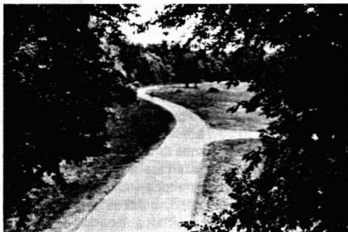
Figure 4.2 Example of bicycle facility continuity in Davenport, Iowa
