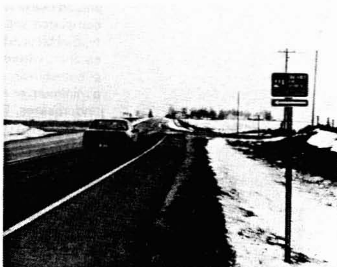
Figure 3.3 Rural Bicycle Lane Facility in Huxley, Iowa
