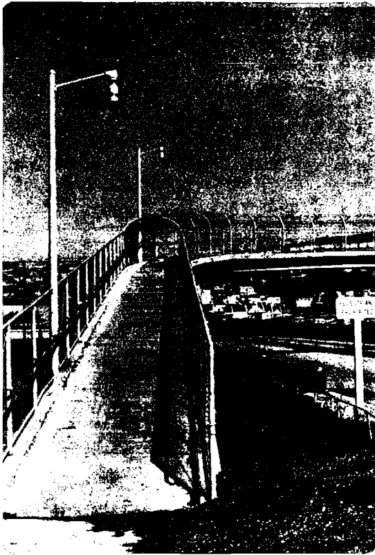
A major bikeway grade separation structure.
