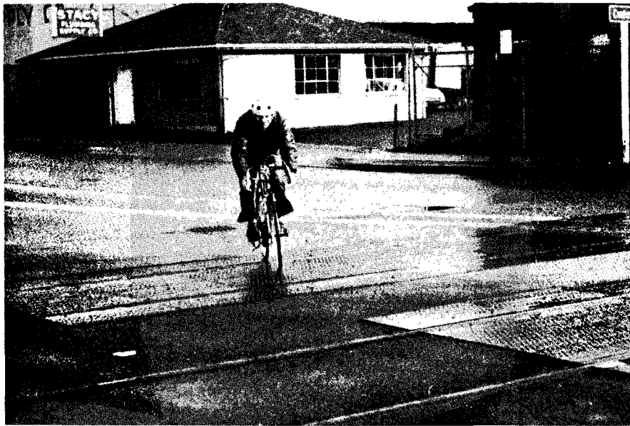
Figure VI-35 RUBBERIZED RAILROAD CROSSING Tacoma, Washington
