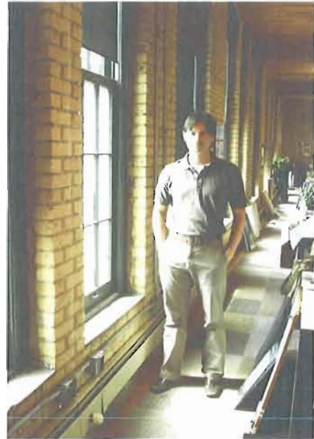
Figure 4.1 Office 3: Low window with handle and sill located approximately 18” from the floor. An employee stands next to the window for scale.
