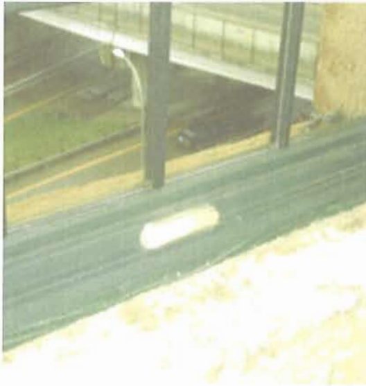
Figure 4.4 Office 3: Handle on 6th floor retrofitted double-hung, double-glazed awning window.
