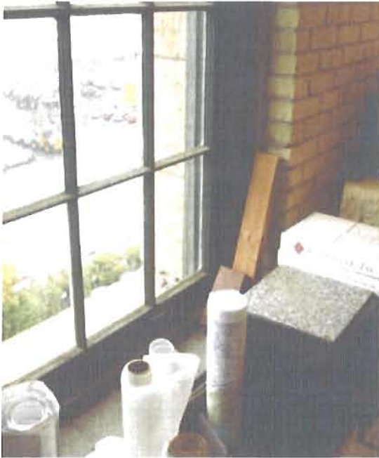
Figure 4.20 Office 3: Used Window. Physical traces indicate that this window does get used, as evidenced by the wood and brick blocking to hold the window open. At the same time, there is some accumulation of items in front of the window, which could potentially hinder window use.
