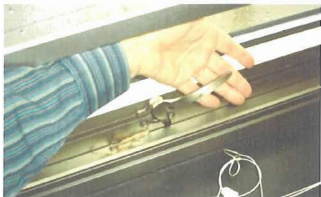
Figure 4.6 Office 1: Lever mechanism on awning window also had mostly positive reports.
