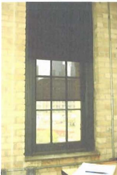
Figure 4.26 Office 3 window shades are a double system for better control of glare and heat on the southwestern side the office space.
