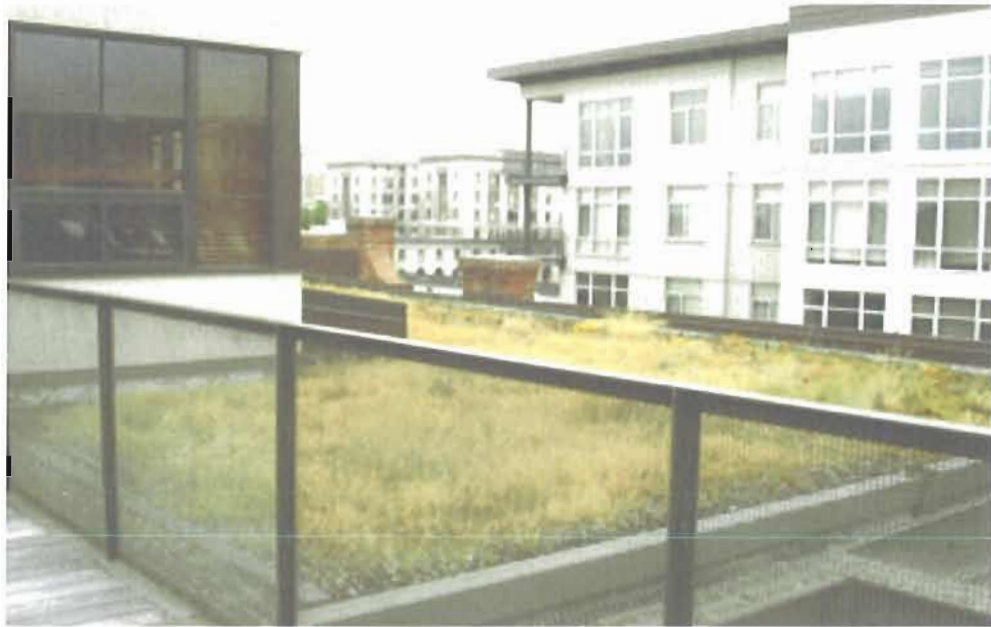
Figure 5.1 Window accessibility from an upper roof garden or deck can still offer potential access to upper level windows, producing similar concerns as that of having windows open to the ground floor. The windows on the far left of the photo are part of an office space.
