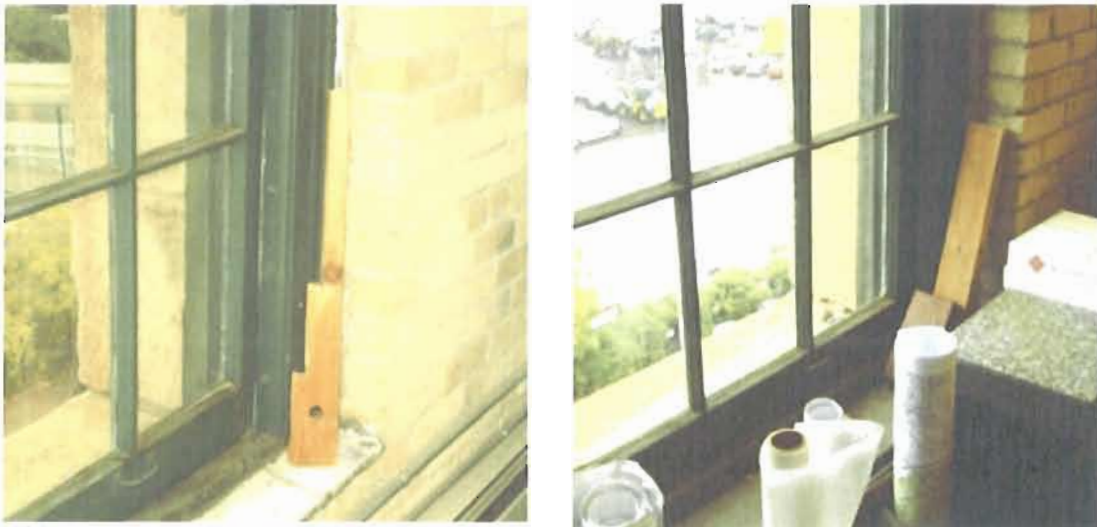
Figure 4.8 (left) and 4.9 (right) Office 3: Props to hold double-hung windows open at different heights reveals use but may indicate that the windows no longer hold themselves open.
