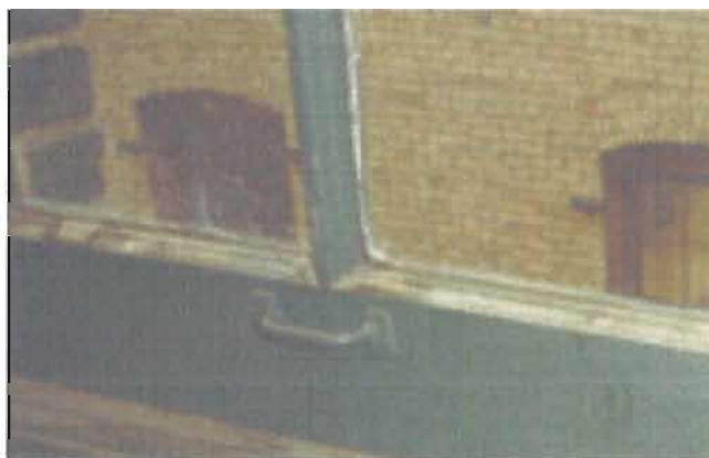
Figure 4.3 Office 3: Handle from original 1886 double-hung window with metal handle.
