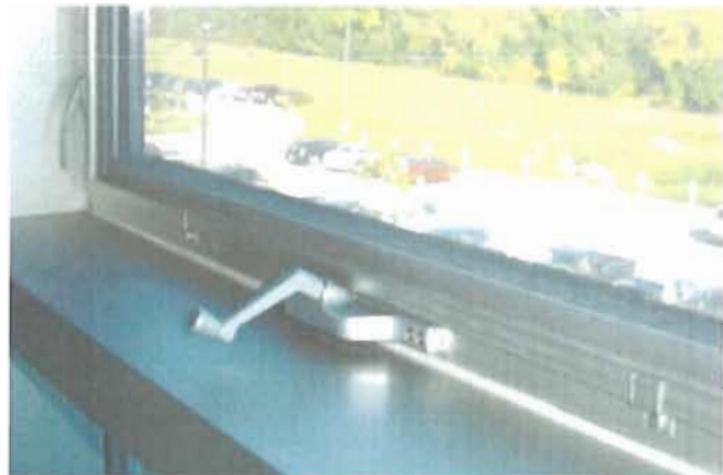
Figure 4.5 Office 2: Crank mechanism on awning window had highest reports of “easy to use” when referring to the crank.
