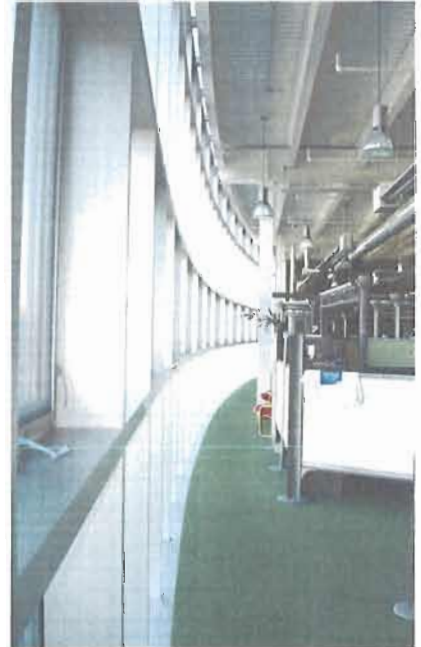
Figure 4.15 (right) Office 2: North Interior The walkway along the window wall (similar on the south wall.)
