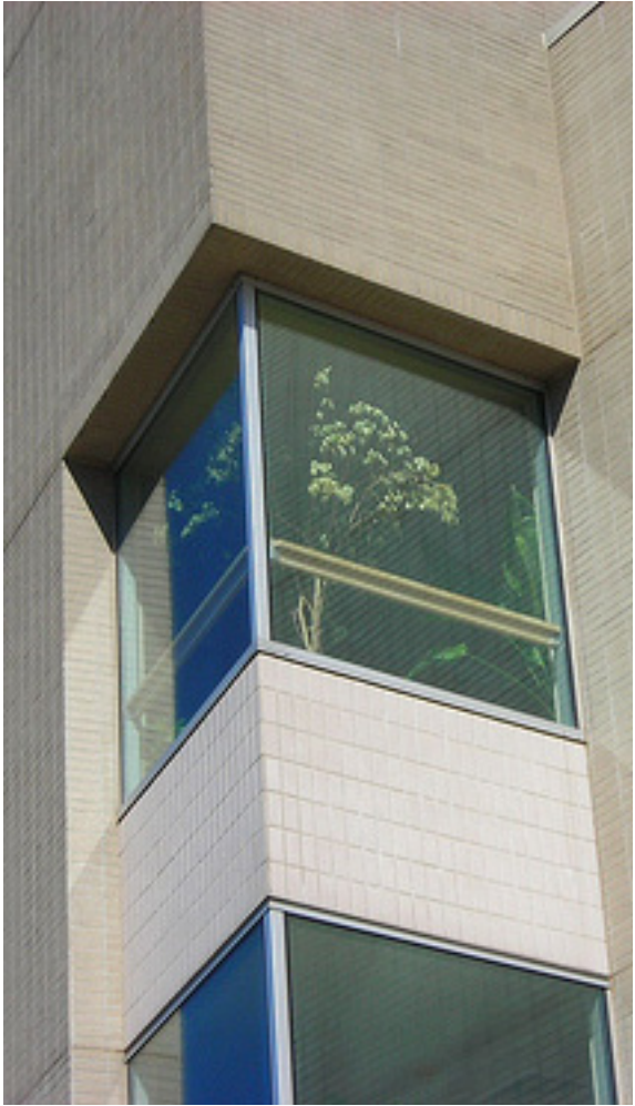
Window detail of elevator lobby
