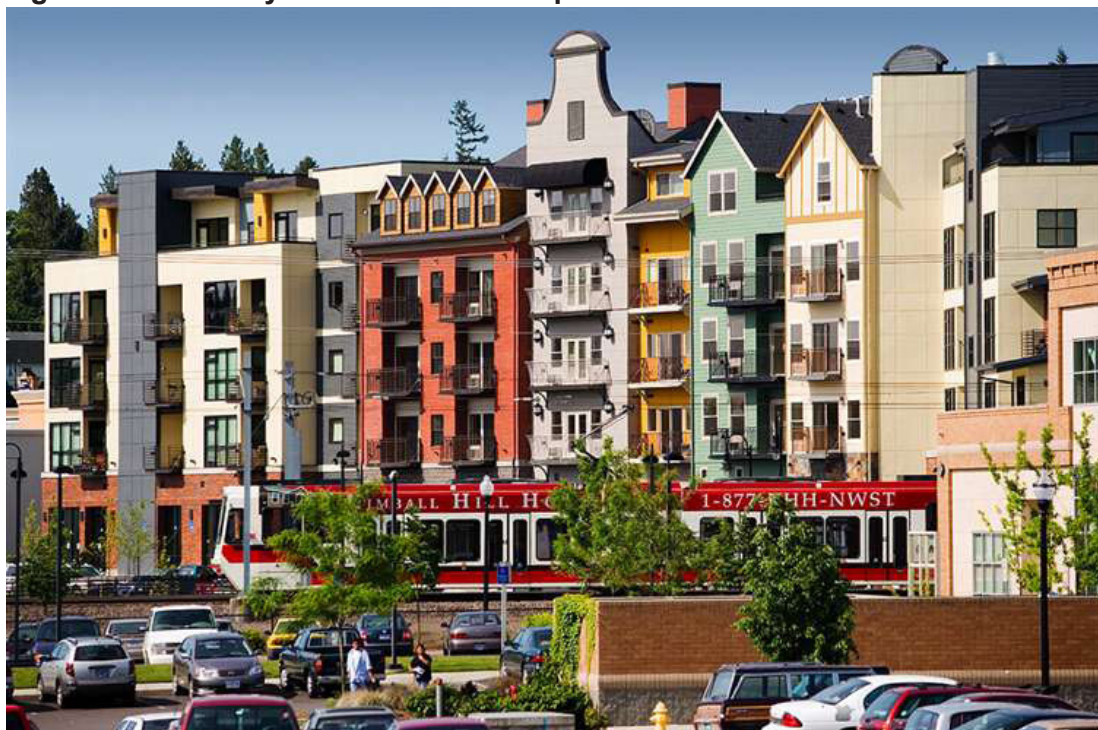
Figure 8 - Multi-story mixed use streetscape in Gresham
