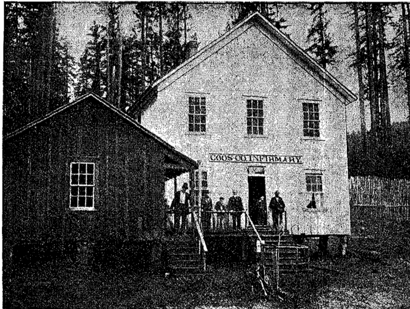
Figure 4.1. “Poor Farm of Coos County,” near Empire City, Oregon, 1892 (an unincorporated community adjacent to North Bend). Coos County had a typical late nineteenth century poor farm for Oregon with a cheaply constructed shack, apparently of box construction with battens for some slight weatherproofing value. The county hospital or “infirmary” was adjacent and slightly more substantial. This cheap construction and limited space was typical of poor farms throughout the country. Even the soon to be maligned “Hillside” farm in Multnomah County was praised more in the First Biennial Report of the [Oregon] State Board of Charities and Corrections (1892) from which this image is sourced.
