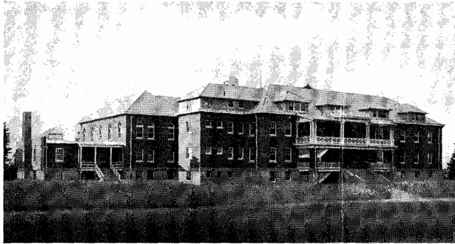
MULTNOMAH COUNTY FARM BUILDINGS AND HOSPITAL, PORTLAND, ORE Roofed with Asbestos "Century" Shingles. Architects BRIDGES & WEBBER, Portland, Ore. Contractors ABBETT TINNING & ROOFING CO.
