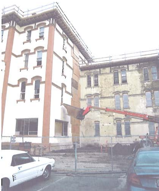
Figure 1.2. State of maintenance during the early phases of rehabilitation at the Oregon State Hospital. The administrative center portion (left and Fig. 1.1) has been repainted during the project, however, the ward wing to the right has had failing windows and peeling paint for many years. Photograph by author.
