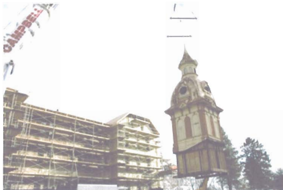
Figure C.4. Removal of the cupola from the “J” building at the Oregon State Hospital in 2009. The cupola was removed for structural analysis and restoration. Courtesy of OSHRP.
