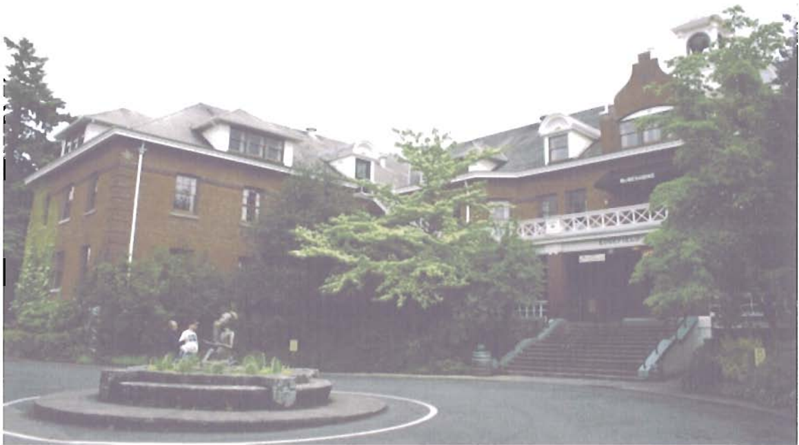
Figure 1.3. Edgefield Manor as photographed in 2010, many years after completion of preservation work. Photo by author.
