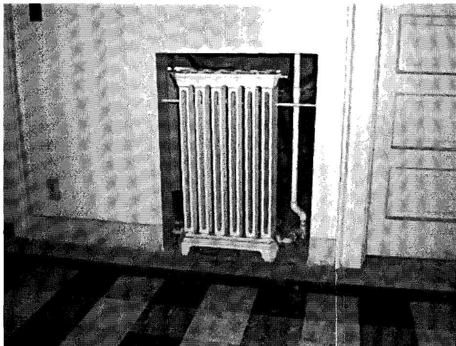
Figure C.6. Typical design of heating system in ward hallway in “J” building. The radiator here is as originally designed. The radiators were placed in cut-outs in the walls between patient rooms and the hallway allowing for maximum heating efficiency, but eliminating any sense of privacy. Photo by Carol Chin, 2008.
