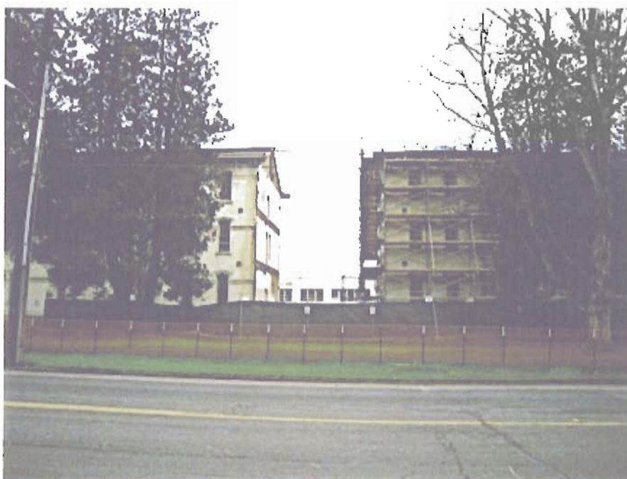
Figure 5.6. State of demolition at the OSH in February 2010, looking to the south. The missing section of building was demolished to separate the portion of the building to be rehabilitated (right and west) from the portion still housing the secure forensic patient ward (left). The portion at left will be demolished when the first phase of construction of new facilities is completed in 2011. Detail in Appendix C. Photo by author.
