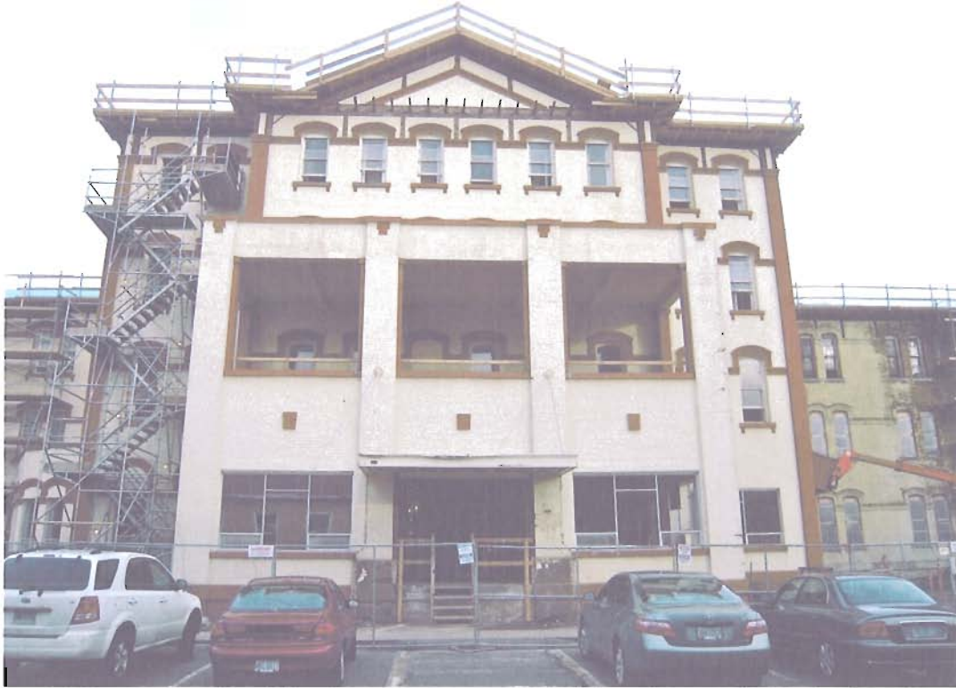
Figure 1.1. Oregon State Hospital's main entrance at the "J" building. Photographed during the construction and demolition phase of its Replacement Project in February 2010. The cupola had recently been removed for structural inspection and preservation. Photograph by author.
