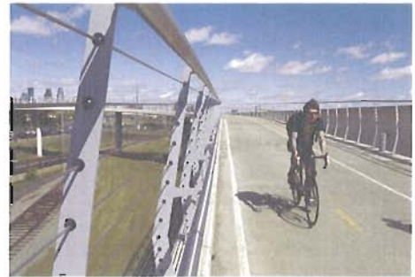
Figure 1-3 Martin Olav Sabo Bridge, Kallusky 2010
