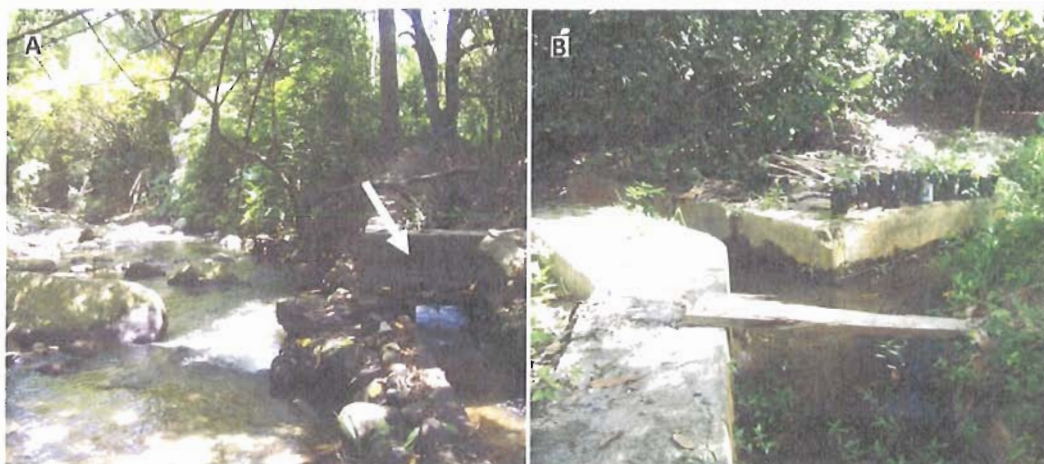
Figure 27. In photo "A" is one Toma of the acequia, the water flows by gravity in the canal where the leader indicates. In photo "B" is the Calicanto or distribution point. Photo by author, August 2009
