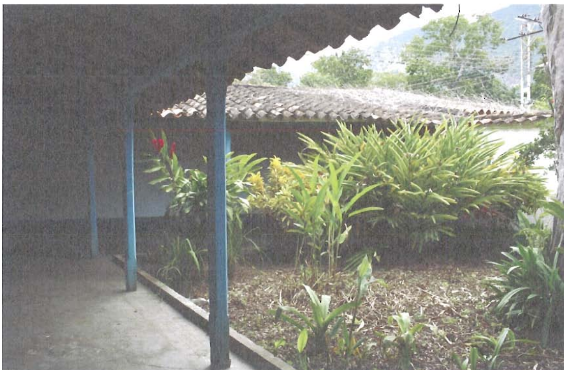
Figure 3. The urban houses are built around interior courtyard, as is this house in Choróní, from the Machado Family. There is usually only one door for residences and many windows on the façade, however, all the rooms face the corridors in the patio or courtyard. Photo by author, August 2009
