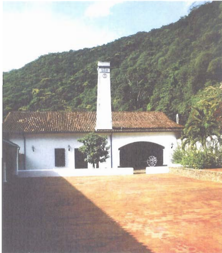
Figure 5. Drying patios for coffee production in sugar cane Haciendas. Observe the tower of the trapiche. House of Hacienda La Vega, Caracas. Photo by Graziano Gasparini from the book Hacienda Houses
