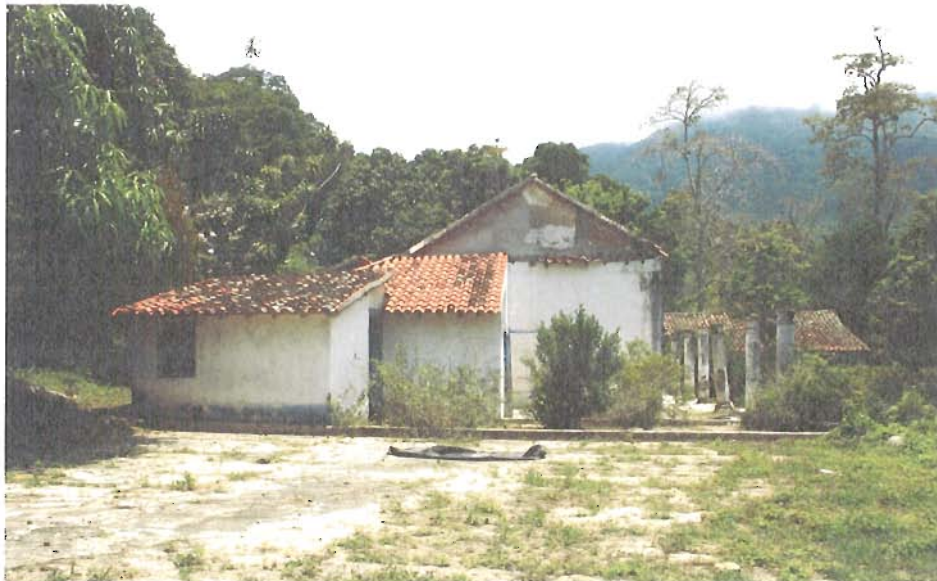
Figure 51. The main house of Hacienda Torres. View from the north patio. This was originally the residential wing. The desbabadero is at the left, as a late addition. Beyond on the right is the two story building originally for storage. Photo by author, August 2009
