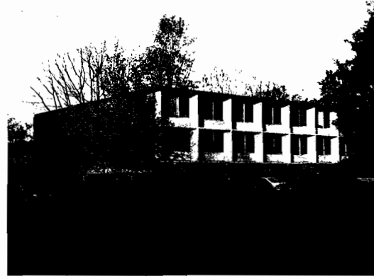
Exterior Photo: Looking Northeast Photo by Author
