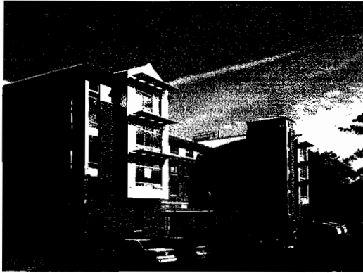
Exterior Photo: Looking Northeast Photo by Author
