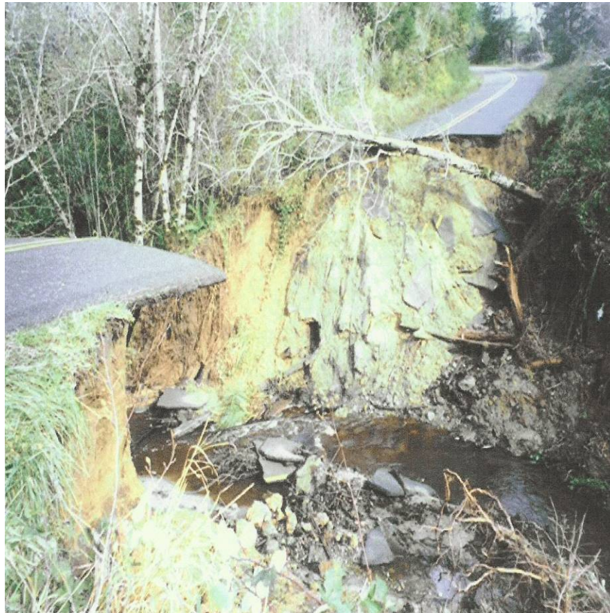
Figure 1. Bill's Creek Road – 30 ft Deep Washout, November 1996, caused flooding in Ferry Creek in Old Town Bandon.
