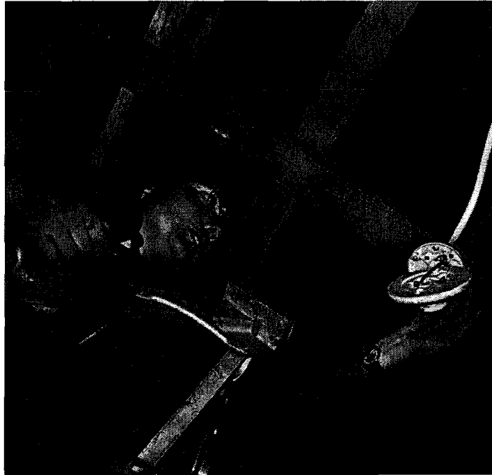
“installing electricity in the barn at Golden” – 1977
