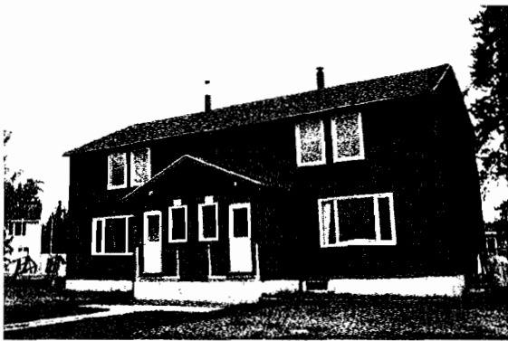
Figure 20: An example of an asbestos shingle clad duplex that retains a high degree of integrity. Photo by the author, August 2009.
