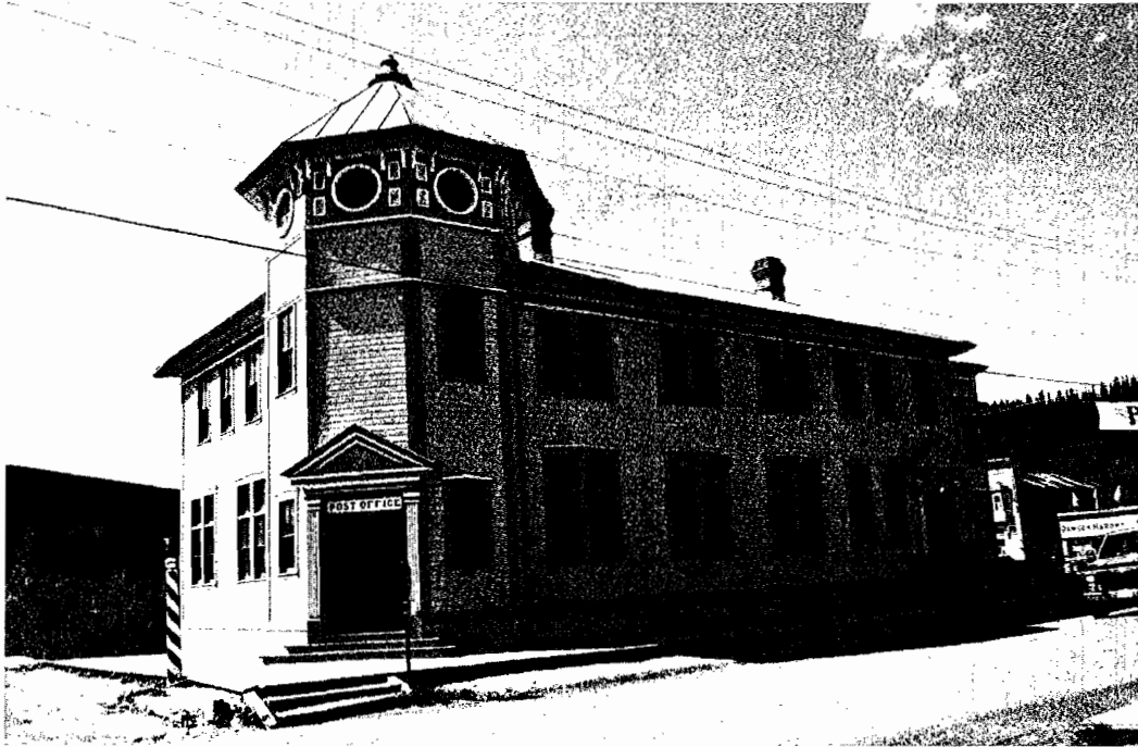
Figure 12: The Old Post Office is the only known architect designed building in the Downtown Character Area. Photo by the author, June 2010.
