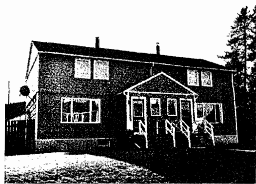
Figure 21: An example of bevel and cedar shingle clad duplex that retains a high degree of integrity. Photo by the author, September 2010.
