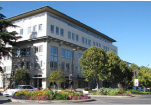
Figure 30: Planted median at Castro Street
