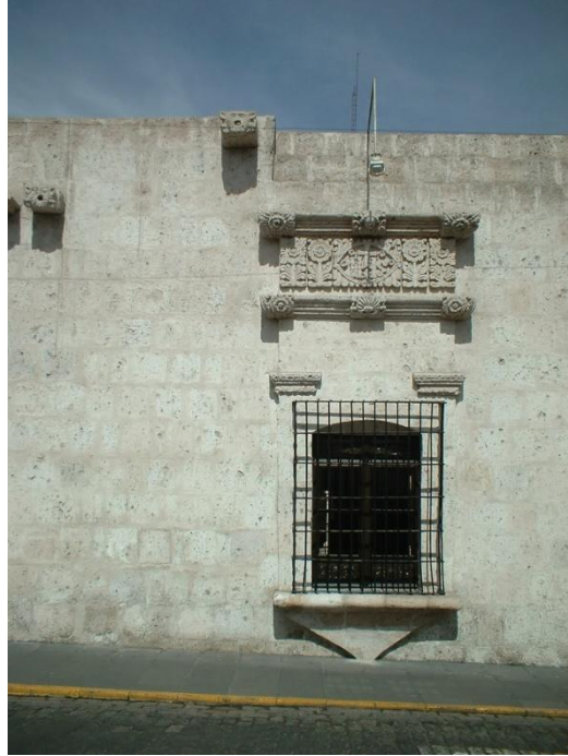
Figure 17. Window opening in Casa del Moral façade. Photograph by author.
