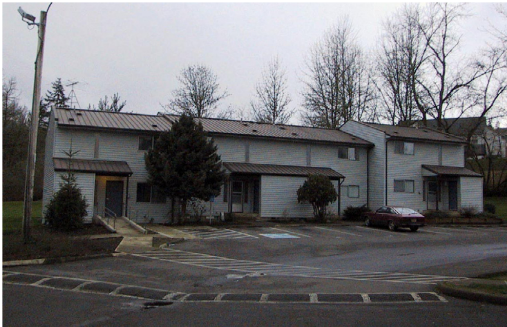
Figure 11: Image of the exterior of existing housing on Glen Creek site, taken from the parking area.
