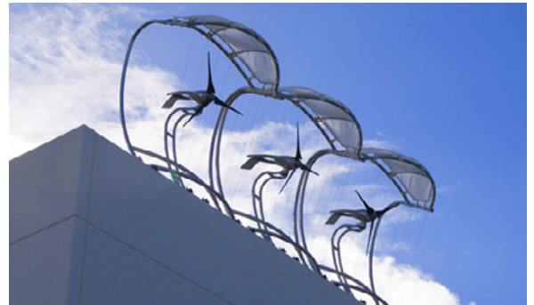
Figure 46: Architectural microturbines are easily scalable for the urban environment. Source: http://inhabitat.com/architectural-wind-modular-wind-turbines/
