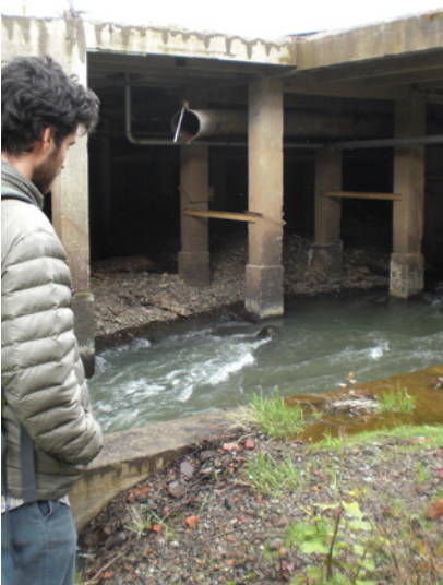
Figure 10: Student observing foundation of former building spanning Pringle Creek.
