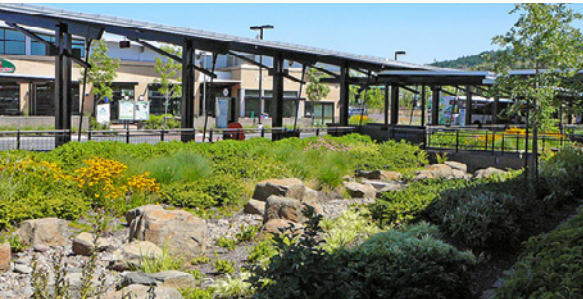
Figure 33: Example of bioswale. Source: http://homemadewilderness.com/2010/03/19/plant-selections-for-bioswales-and-rain-gardens/
