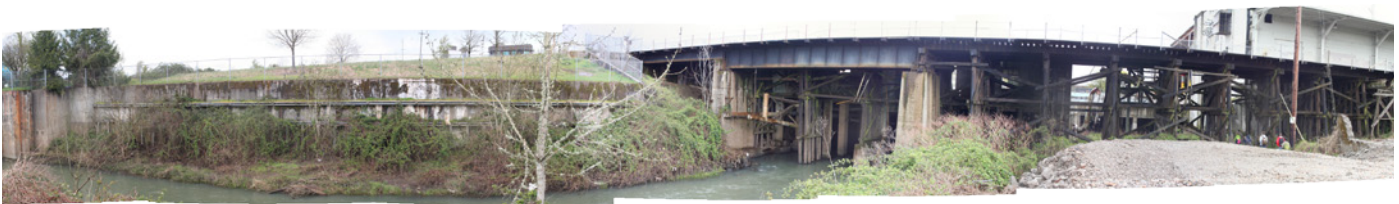
Figure 28: Retaining wall along the north bank of Pringle Creek.
