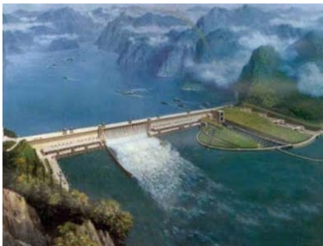
Three Gorges Dam in China
