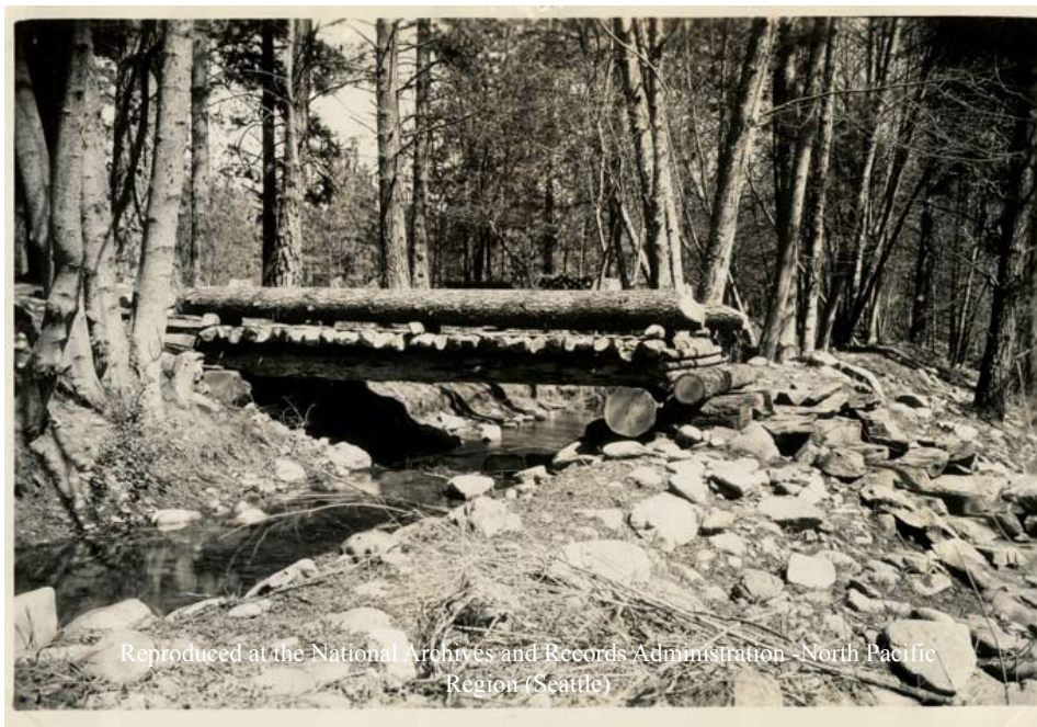
Figure 112. Photograph No. 34; “McKee Bridge Forest Camp, foot-bridge across irrigation ditch”; 1936, Records of the U.S. Forest Service, Record Group 95, Photographs, Applegate Ranger District, Box 73, V-1, Forest Service Projects and Activities (through World War II), National Archives and Records Administration–North Pacific Region (Seattle).
