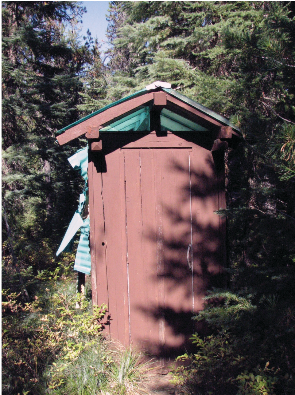
Figure 180. Camp toilet, constructed from the 1945 Recreation Plans Handbook. This one has corrugated plastic roofing, damaged from the winter. Both shingle and plastic roofing are appropriate, and were indicated in original construction plans.
