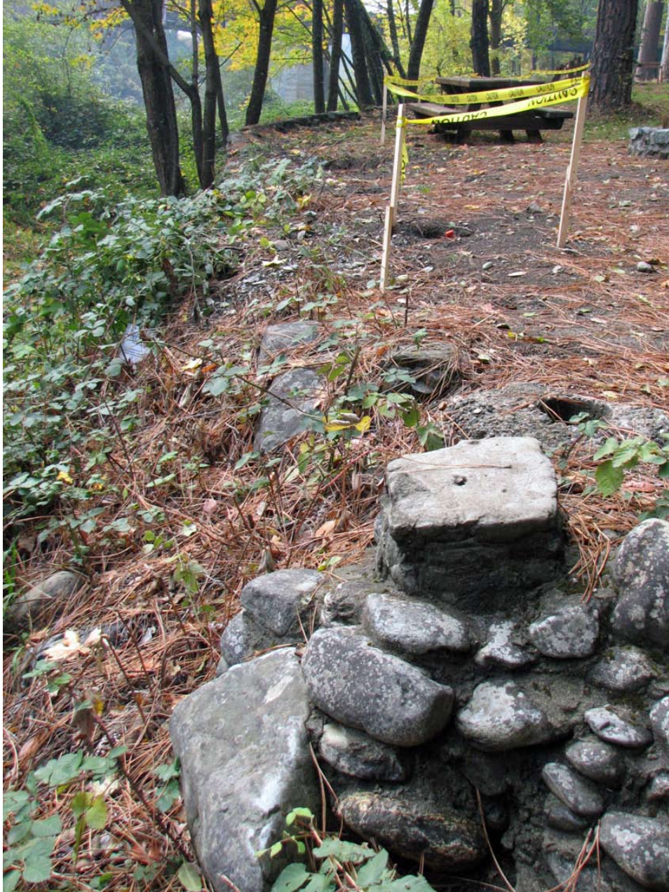
Figure 94. Former fence supports atop river wall. These fences have been replaced.
