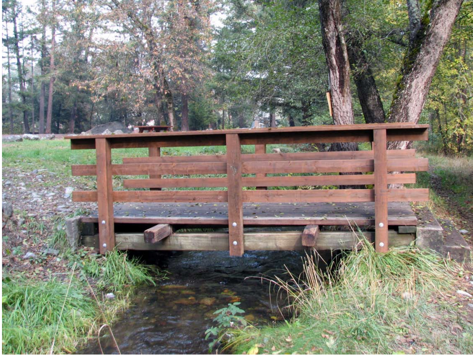
Figure 87. Modern bridge that replaced historic type.
