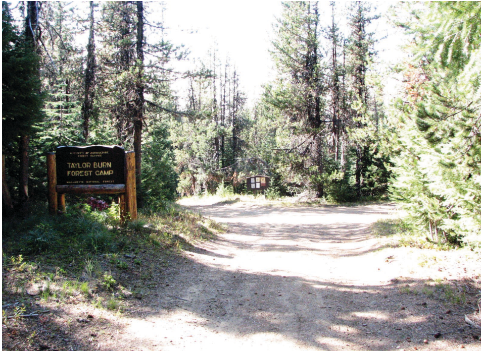
Figure 164. Forest Camp entrance. The sign was rehabilitated in 2001, and was constructed from the 1930s Forest Service Recreation Plans Handbook, Plate 13-A, Design B.
