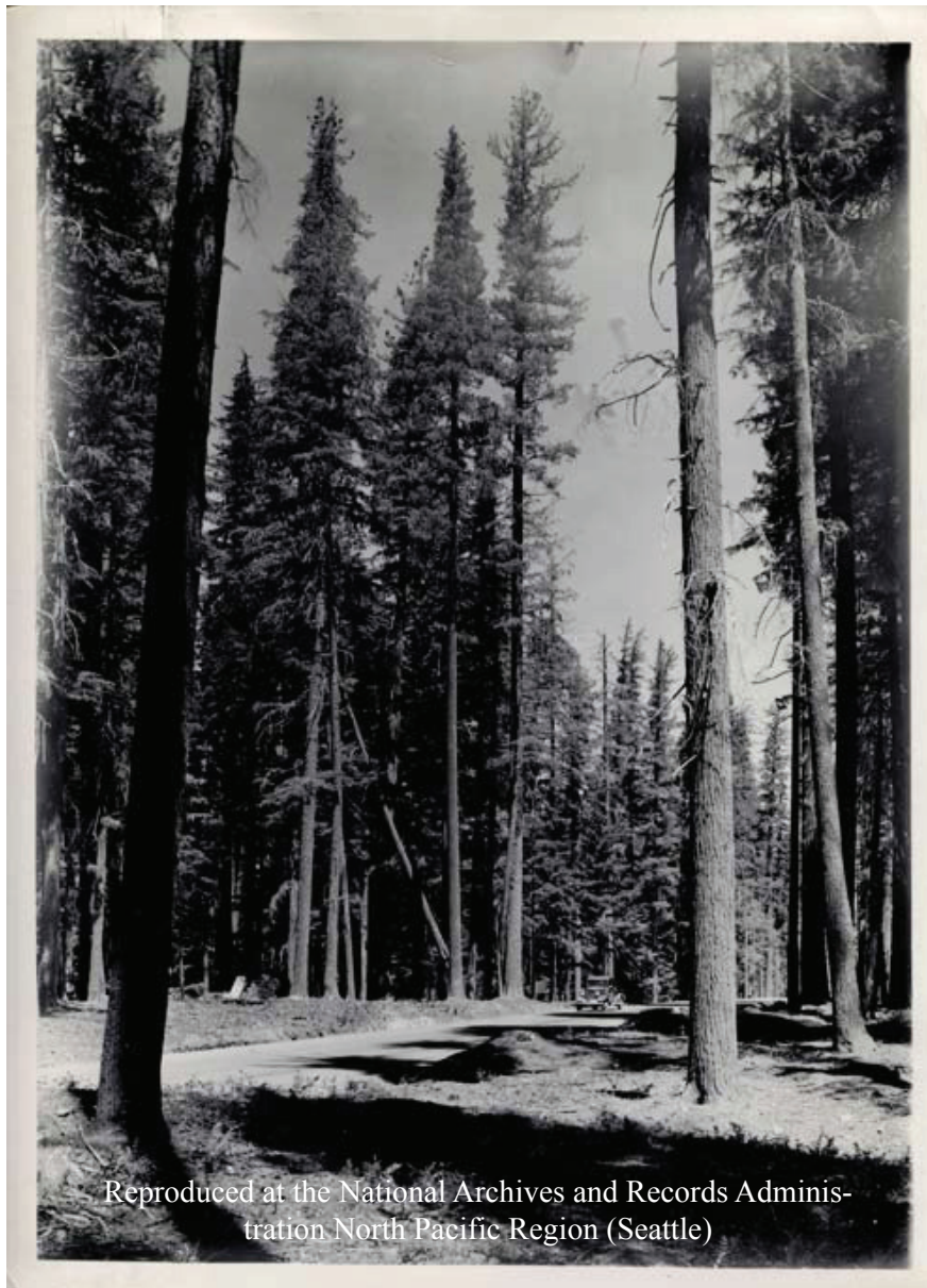
Figure 150. Photograph No. 11; “Crater Lake Road, shows truck traveling on new grade near Union Creek”; 1935; Records of the U.S. Forest Service, Record Group 95, Rogue River National Forest, Box 80, Y-1, Forest Service Projects and Activities (through World War II), National Archives and Records Administration–North Pacific Region (Seattle).
