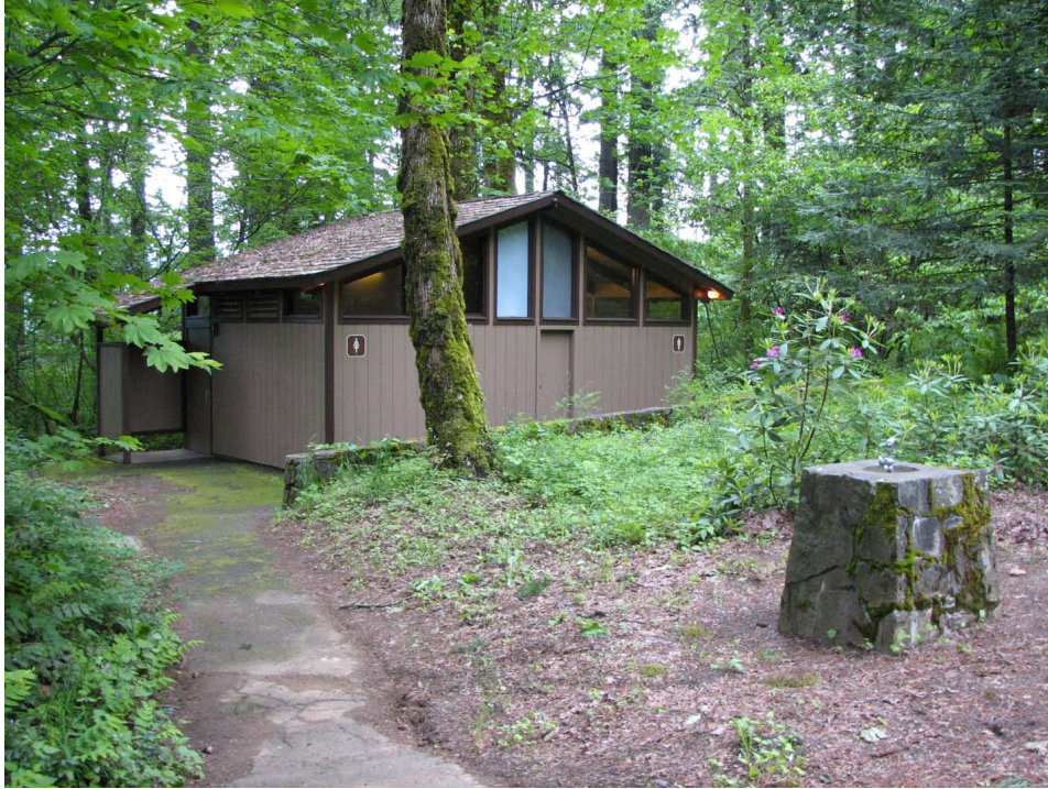
Figure 16. More modern campground restroom, date of construction is unknown. In the foreground, the water dispenser appears to date from the Civilian Conservation Corps period (however, these did not appear on any plans). Further research is needed on the water dispensers, and the rock retaining wall just in front of the restroom.
