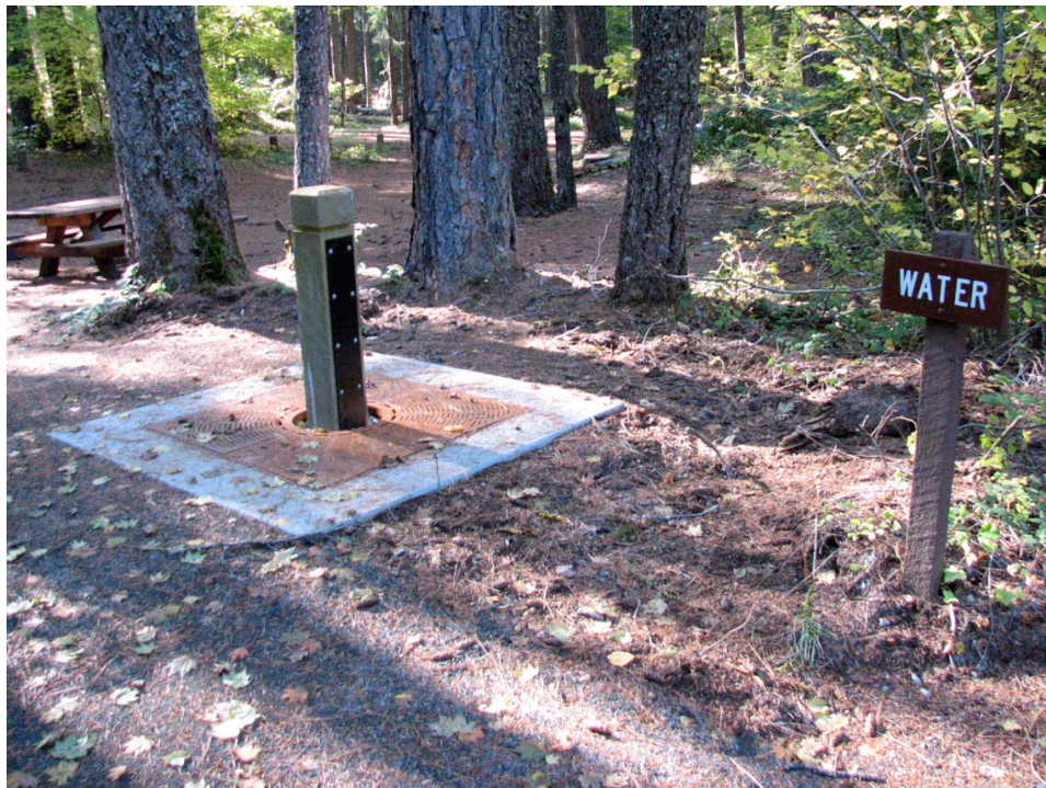
Figure 132. New water system infrastructure and sign. This new design is appropriate, as it clearly demonstrates distinctive decorative characteristics, yet also demonstrates new construction, distinguishing it from Civilian Conservation Corps improvements.
