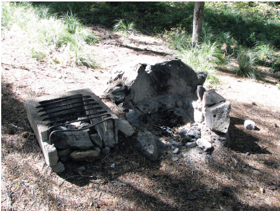
Figure 169. Civilian Conservation Corps-era rustic stove, with 1950s concrete stove added later. The concrete stove was constructed from the 1945 Recreation Plans Handbook.
