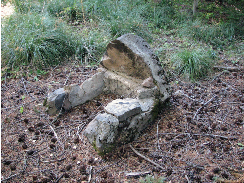
Figure 170. Civilian Conservation Corps rustic stove, constructed of local volcanic rock. Concrete inserts were added to protect the rock from quick disintegration.
