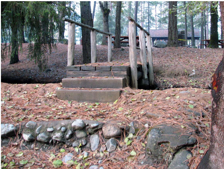
Figure 88. Historic cobble steps, showing erosion.
