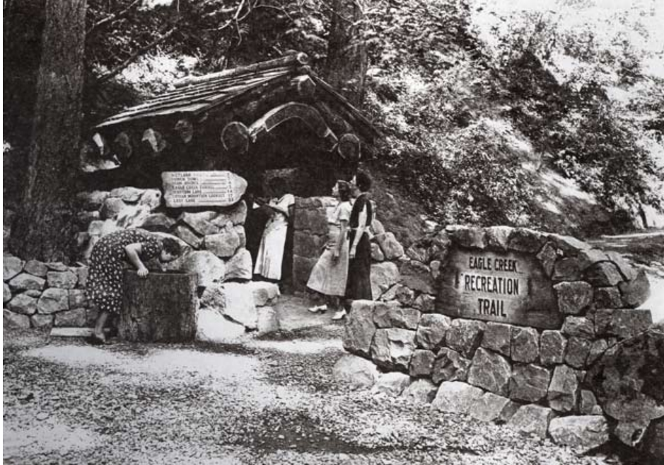
Figure 64. Civilian Conservation Corps improvements at Eagle Creek Forest Camp. Shown is the rustic hiker register, rock wall, and Eagle Creek Recreation Trail sign. Courtesy USDA Forest Service, Heritage Files, Columbia River Gorge National Scenic Area, Hood River, Oregon.
