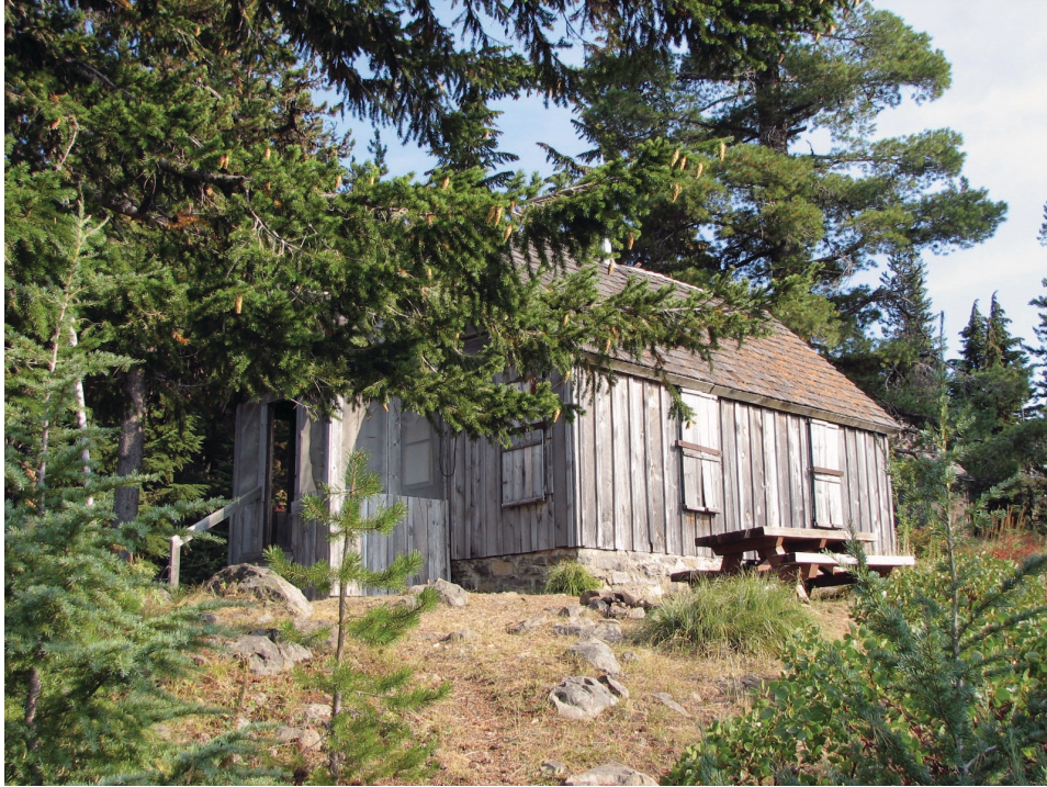
Figure 183. Taylor Burn Guard Station. At some point between 1940 (the date the station was moved to this location) and the present, the front porch has been enclosed, and the horizontal clapboards replaced with board and batten siding.
