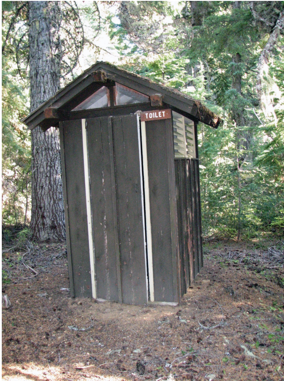
Figure 179. Camp toilet, constructed from the 1945 Recreation Plans Handbook. This one has a wooden shingle roof.
