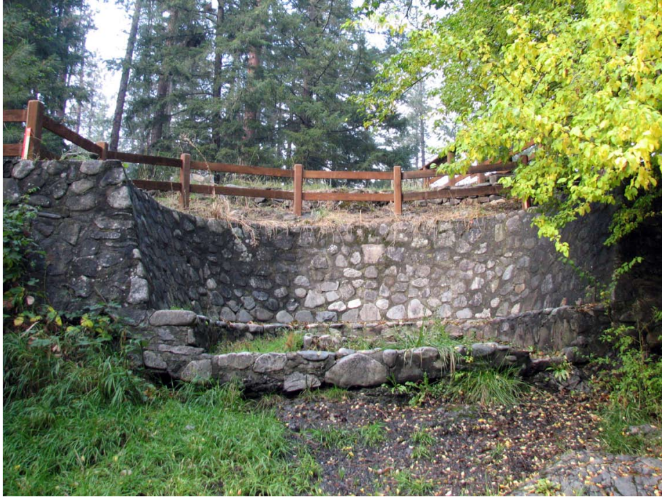
Figure 97. Barbeque pit, showing undercut that must be repaired.
