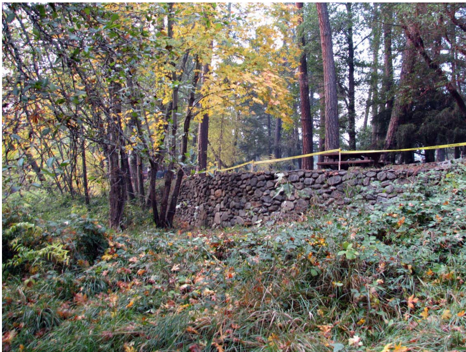
Figure 90. Civilian Conservation Corps era rustic wall along Applegate River.
