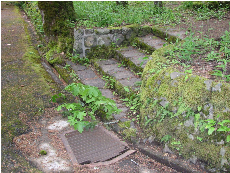
Figure 54. Lower area rustic rockwork and drain.
