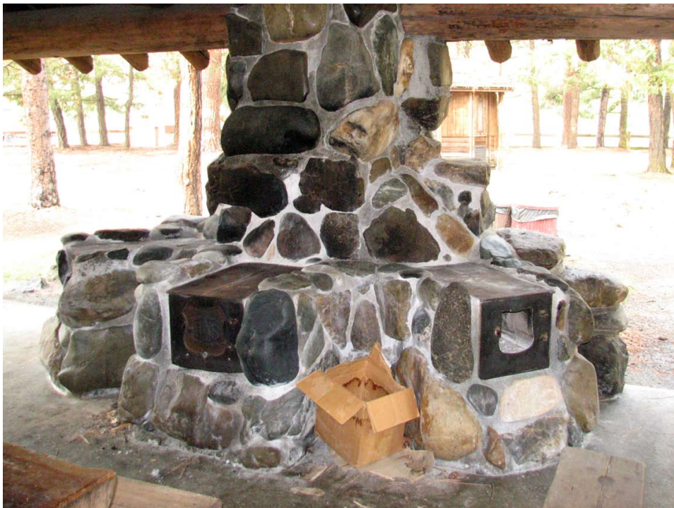
Figure 82. Community kitchen shelter stove, rehabilitated for use.
