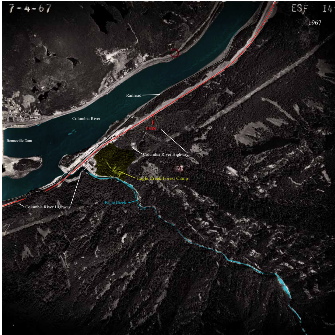
Figure 11. 1967: Along this portion, the existing section of U.S. 30 will become the eastbound lane of I-80N, while the westbound lane is being constructed on the north side of the railroad bridge (closest to the river). The most noticeable element here is that the Columbia River Highway road alignment is becoming more difficult to see. Aerial photograph courtesy of the University of Oregon Map and Aerial Photography Library at Knight Library.
