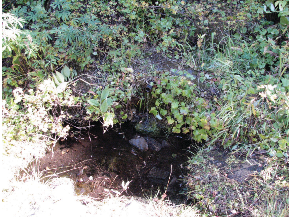
Figure 177. Spring, showing concrete retention wall and embedded pipe.
