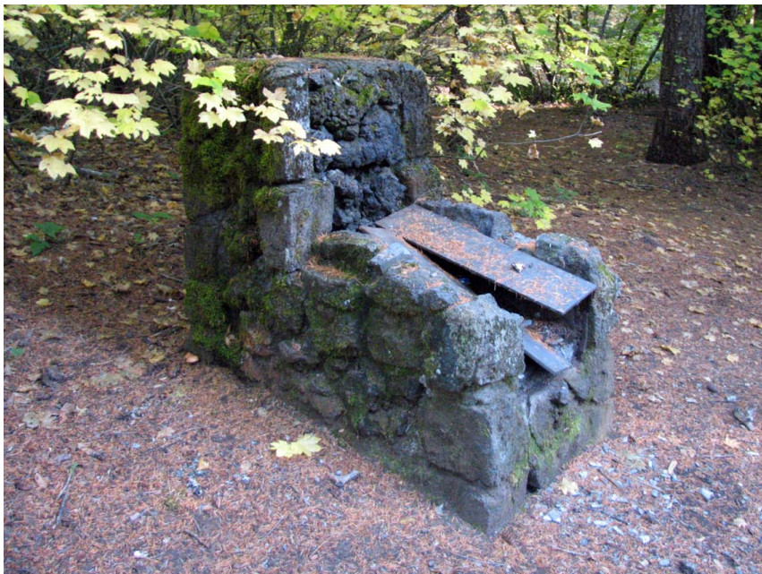
Figure 137. Historic Civilian Conservation Corps rustic camp stove, firebox in poor condition.
