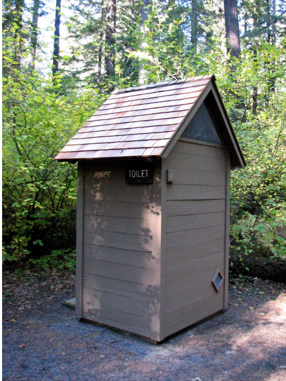
Figure 138. Historic toilet, constructed from the 1930s Recreation Plans Handbook design, Plate II for “R-6 Standard Single Toilet”.
