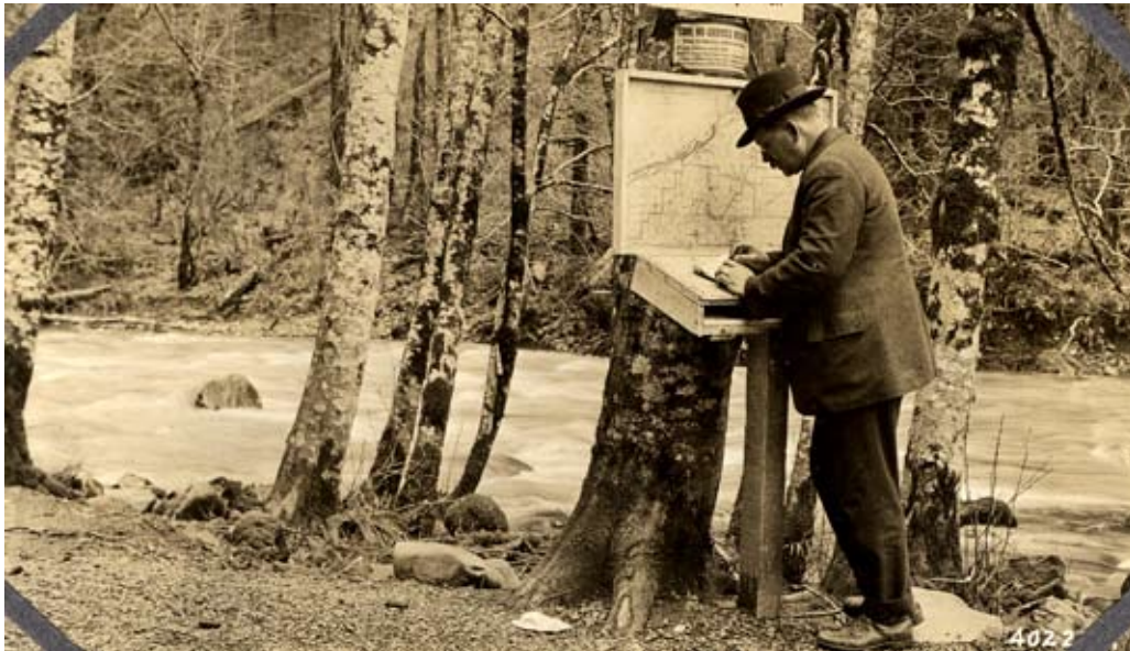
Figure 57. July 1916: First hiker register booth constructed at the Eagle Creek Forest Camp. Courtesy USDA Forest Service, Heritage Files, Columbia River Gorge National Scenic Area, Hood River, Oregon.
