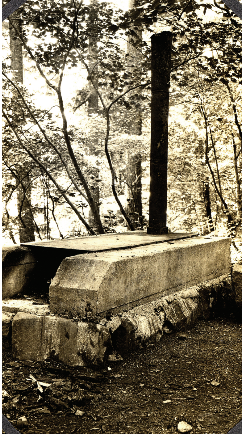
Figure 60. 1923: Utilitarian camp stove design constructed at the Eagle Creek Forest Camp, 1916. Courtesy USDA Forest Service, Heritage Files, Columbia River Gorge National Scenic Area, Hood River, Oregon.
