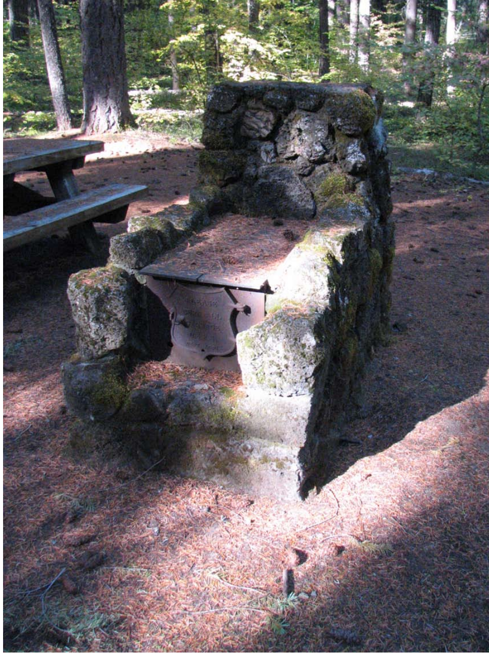
Figure 135. Historic Civilian Conservation Corps rustic masonry stove, more refined design example.
