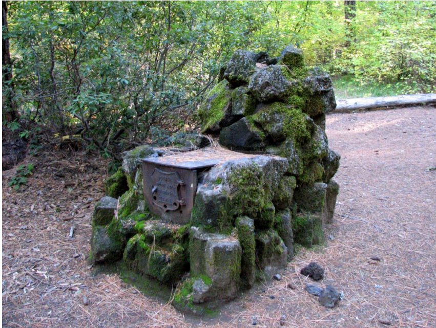
Figure 136. Historic Civilian Conservation Corps rustic masonry stove, irregular cobble design example.
