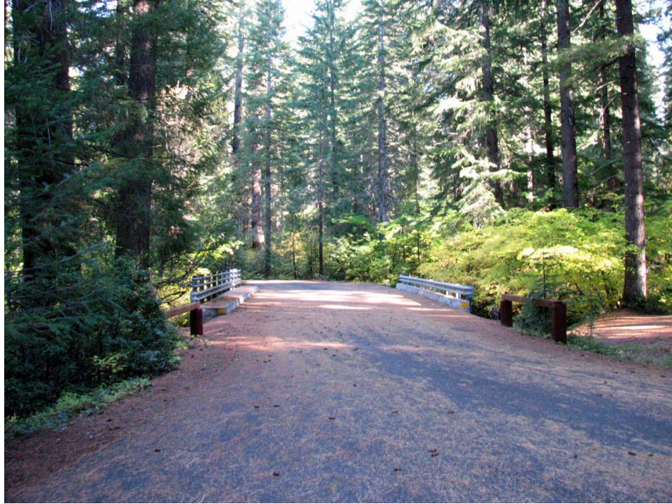
Figure 127. Bridge across Union Creek, constructed in 1963.
