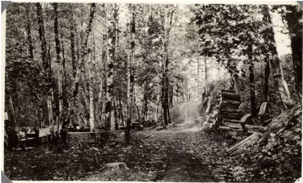
Figure 56. Eagle Creek Forest Camp general scene, taken between 1916-1936. Given the road slope, the vegetation to the left, and the sharp hillside to the right, this picture was likely taken where the lower road and parking area exist immediately along Eagle Creek today. Courtesy USDA Forest Service, Heritage Files, Columbia River Gorge National Scenic Area, Hood River, Oregon.
