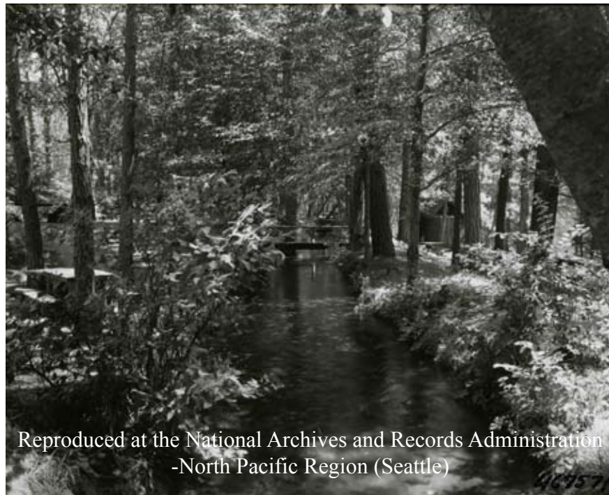
Figure 111. Photograph No. 33; “McKee Bridge Forest Camp, foot-bridge across irrigation ditch”; 1936, Records of the U.S. Forest Service, Record Group 95, Photographs, Applegate Ranger District, Box 73, V-1, Forest Service Projects and Activities (through World War II), National Archives and Records Administration–North Pacific Region (Seattle).
