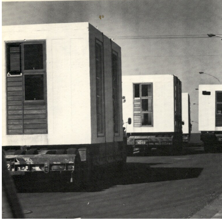
Figure 19: Kurokawa, trucks transporting concrete capsules for Concrete Capsule House, 1975
