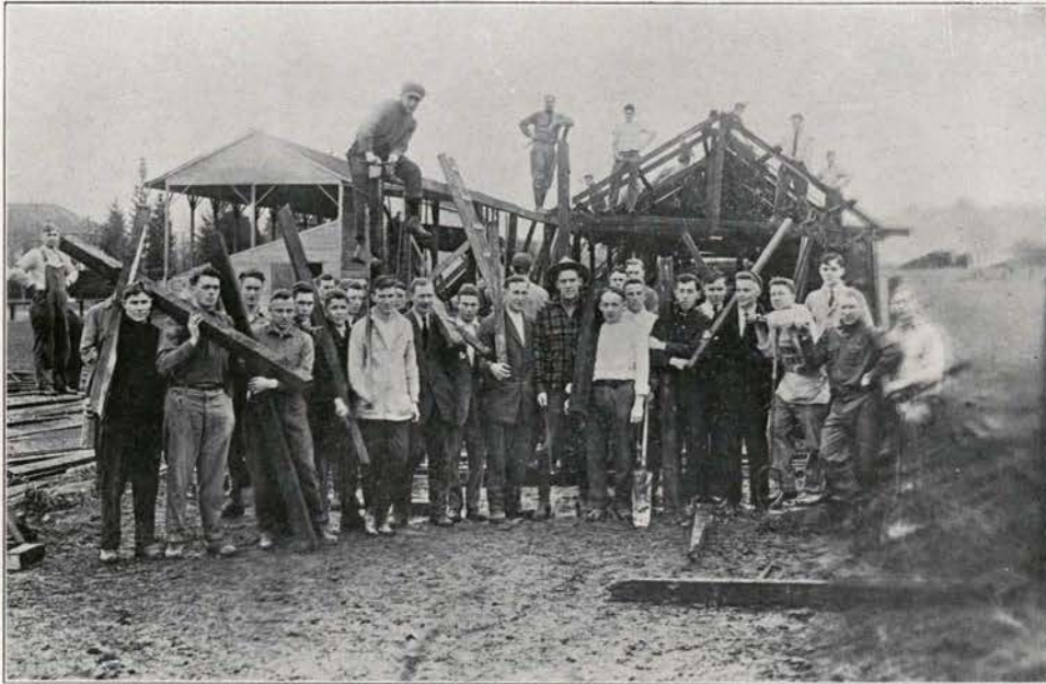
Annual Rebuilding of Running Shed
