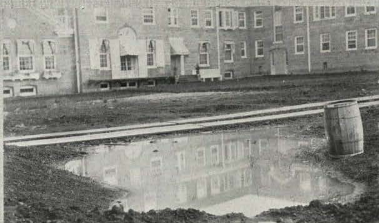
And an open air swimming pool and board walk ***
