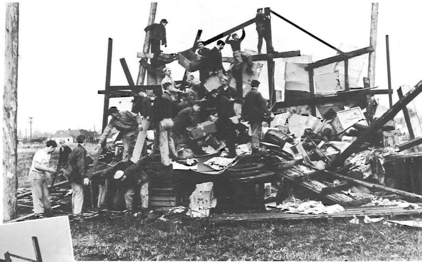
Framework, above, for Oregon's Homecoming bonfire on Twentieth Street sub-marginal lands is swarming with Freshman Class activity. At left, closeup shows that structural engineering plays part in annual pyrotechnic display for graduates.
