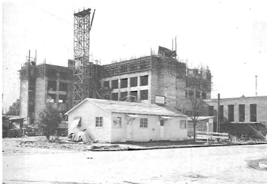
Construction on the new women's dormitory proceeds rapidly during the year, with completion scheduled for next year.
