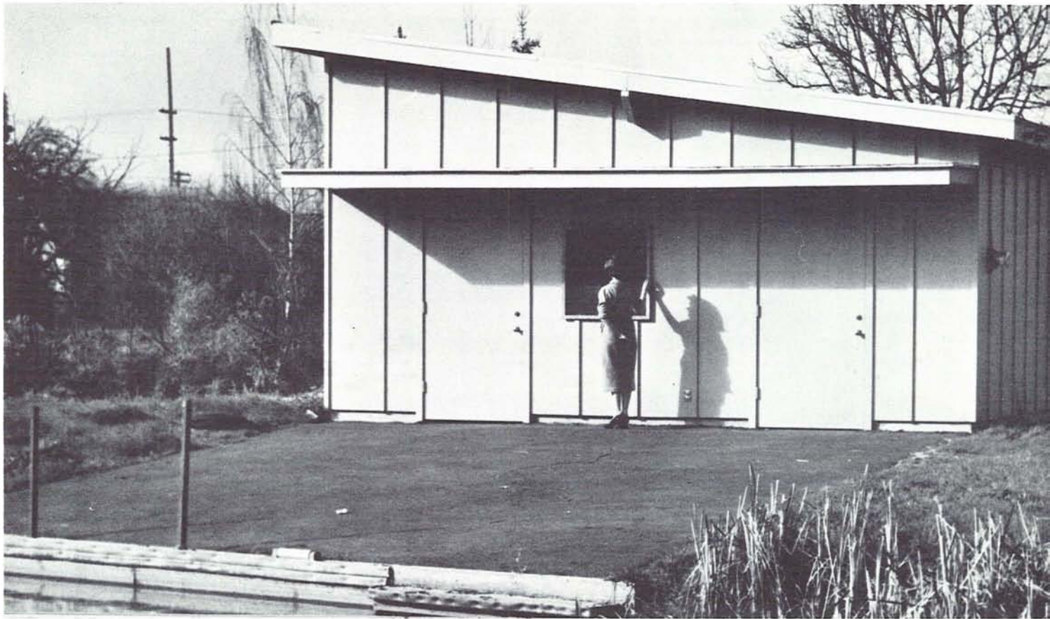
One of the first steps in the Millrace restoration development program was the building of an area where canoes could be stored. The boat house, pictured above, accomplished just that purpose. The black-top launching area and docks provided a convenient starting and finishing place for canoe trips and into the upper "wilderness" area of the 'Race.
