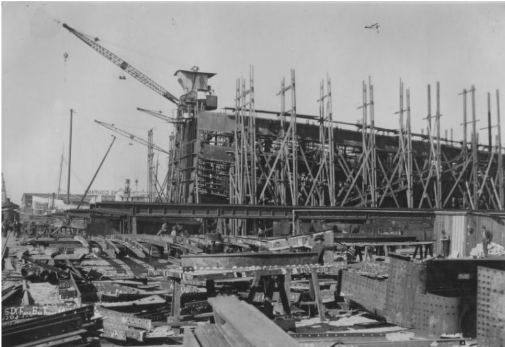
Figure 14: Steel Vessel Under Construction at Union Iron Works, Oakland Inner Harbor. Image courtesy of Bancroft Library, University of California, Berkeley
