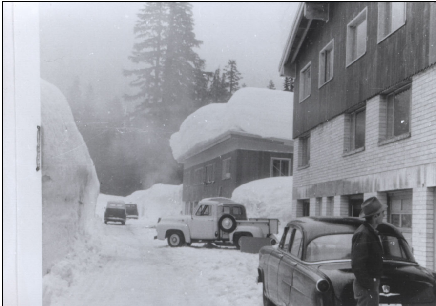
Figure 4-10. Building #227 Duplex Residence during a Crater Lake winter, date unknown. Note the thick snow buildup on the roof. Crater Lake National Park Museum and Archives Collections. Collection 8889 Building and Construction Files.
