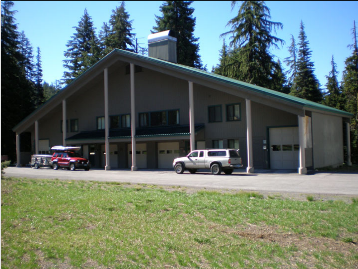
Figure 4-11. Building #227 Duplex Residence, Summer 2010. Only upon close inspection can elements of the building's original design be discerned underneath the new roof and façade treatment.
