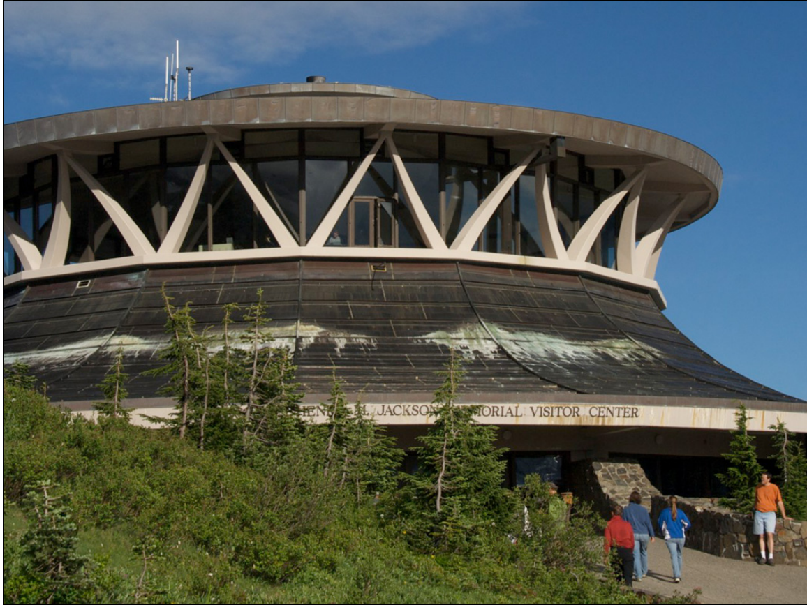
Figure 1-2. The Henry M. Jackson Memorial Visitor Center, Mount Rainier National Park, Washington. Demolished 2009. In 1986 Jonathan Monroe described the building as “One of the worst... buildings in the national park system.” 6 However, this is a “view” expressed without the understanding that the building was purpose designed for day-use skiing activities during the winter months at the park. This use never developed and the purpose of the building changed, leaving it to be used for a purpose it was not designed to fulfill. Photograph by Nathan Vander Wilt, 2007.
