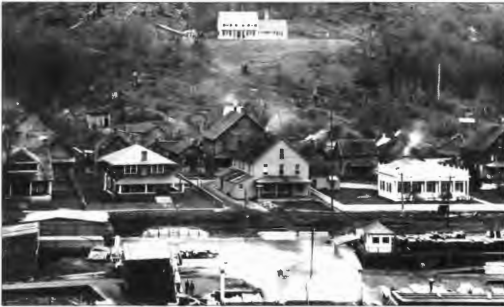
54. McCormick, Lewis County, Washington. This southerly view, c. 1912–15, shows State Highway 6 in the foreground and Lawrence's McCormick Lumber Company office building at the far right. In the distance at the top of the photograph is Lawrence's house for J. E. Wheeler. Between them was built Lawrence's Presbyterian Church (demolished c. 1929), photograph, c. 1915. Lawrence Collection, courtesy of Special Collections, Knight Library, University of Oregon.
