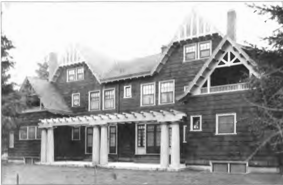
15. E. F. Lawrence House, Portland, built 1906, rear facade, photograph c. 1906. Lawrence Collection, courtesy of Special Collections, Knight Library, University of Oregon.
