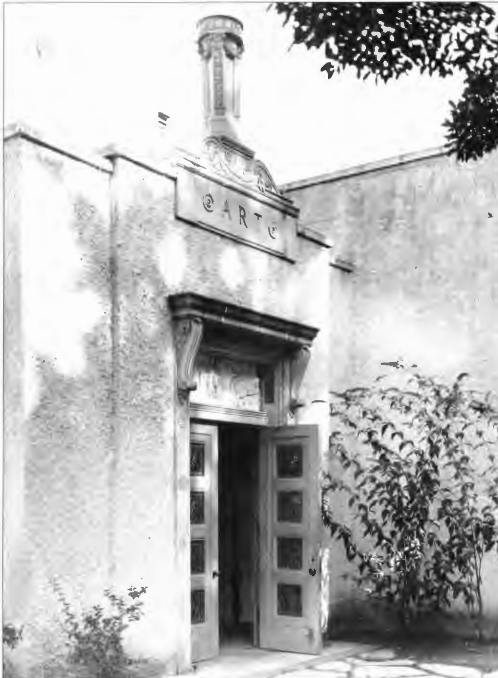
41. E. F. Lawrence, School of Architecture and Allied Arts, University of Oregon, entrance to Arts Wing, photograph c. 1930. Courtesy of University of Oregon Archives.
