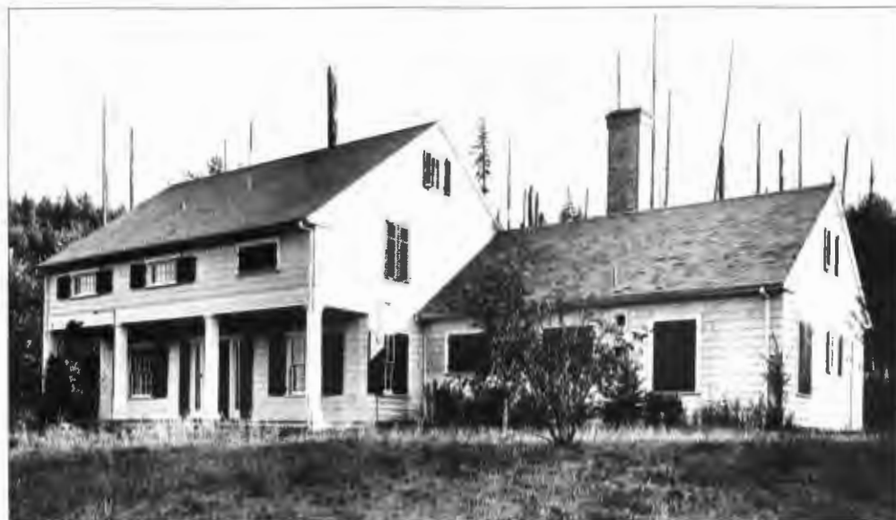
9. E. F. Lawrence, J. E. Wheeler House, McCormick, Washington, built 1912, front facade, photograph c. 1913. Lawrence Collection, courtesy of Special Collections, Knight Library, University of Oregon.
