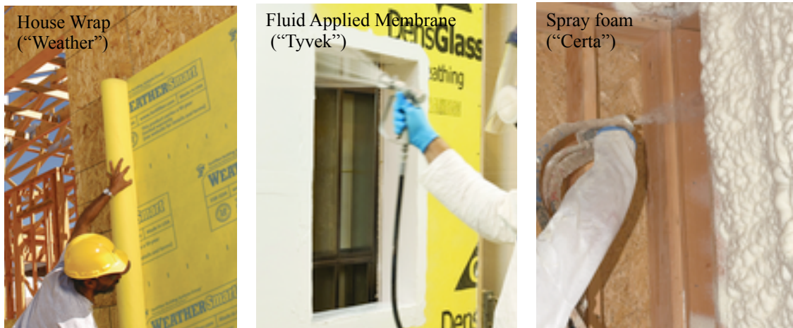
Figure 2.2. Air barrier materials.
